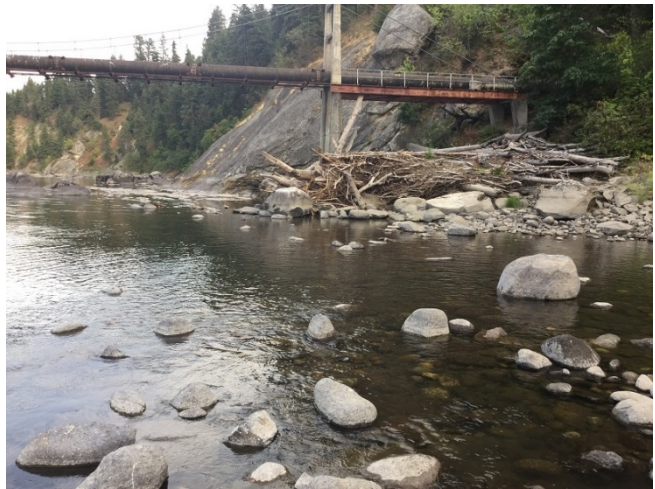
Figure 4-13. Photograph of Rare Log Jam Racked on a Crossing Abutment in Reach 8, near RM 22.8
