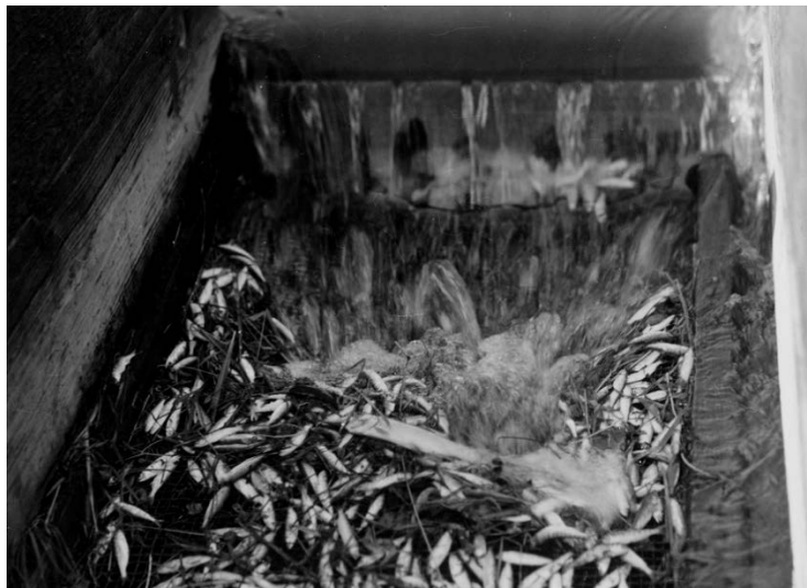
Figure 2-12. Photograph of Dead Chinook Fingerlings in an Unscreened Diversion Box at the End of the Rock Island Branch of Dryden Canal – 1940 (source: Oregon State University Libraries Special Collections & Archives Research Center)
