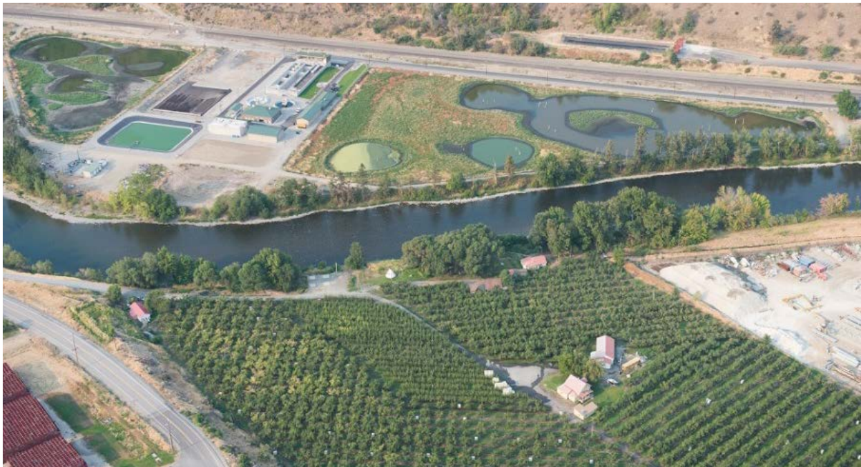
Figure 2-15. Oblique Aerial Photograph of the Sewage Treatment Facility near Cashmere (source: Shane Wilder of Icicle TV, flight provided by Lighthawk and the UCSRB)
