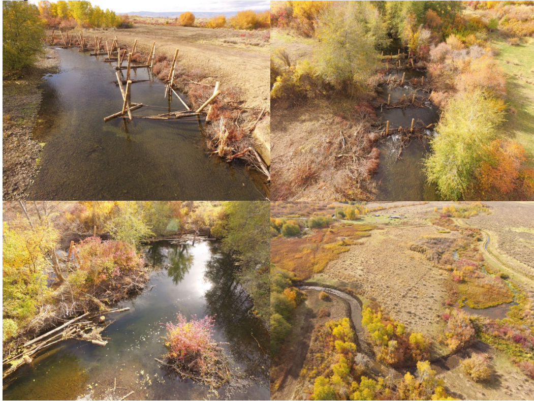
Figure 1. Image depicts restoration work post implementation along Toppenish Creek near river mile 37 (8/8/16-9/2/16). Habitat structures pictured in images above were designed by Natural Systems Design (NSD).
