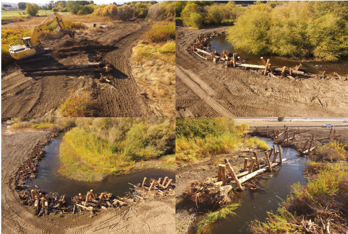
Figure 2. Images depict restoration work during and after implementation (9/6/16-10/14/16). Structures were designed by Natural Systems Design (NSD).
