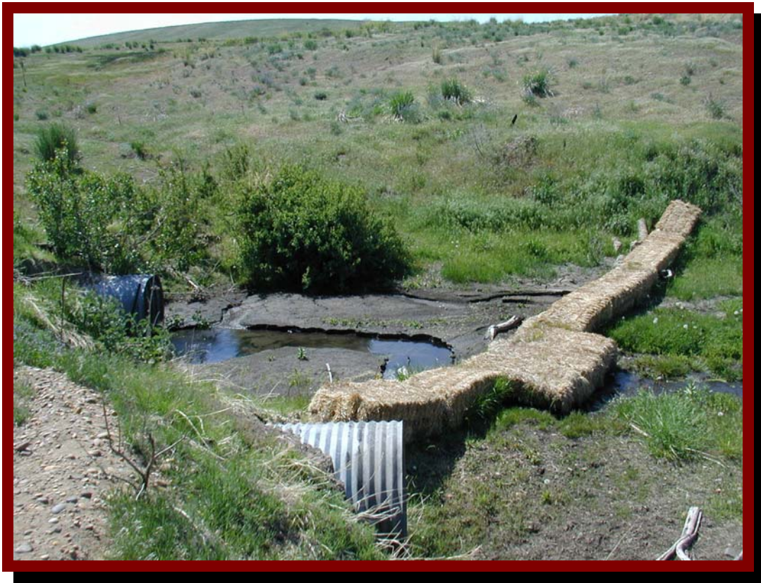
Figure 5. Sediment captured behind a bale structure on headwaters of Mule Creek.
