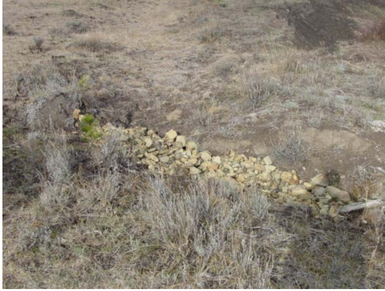
Figure 2. Headcut in cattle trail stabilized with rock structure.
