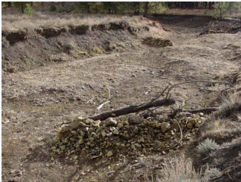
Figure 3. Small rock check structure.
