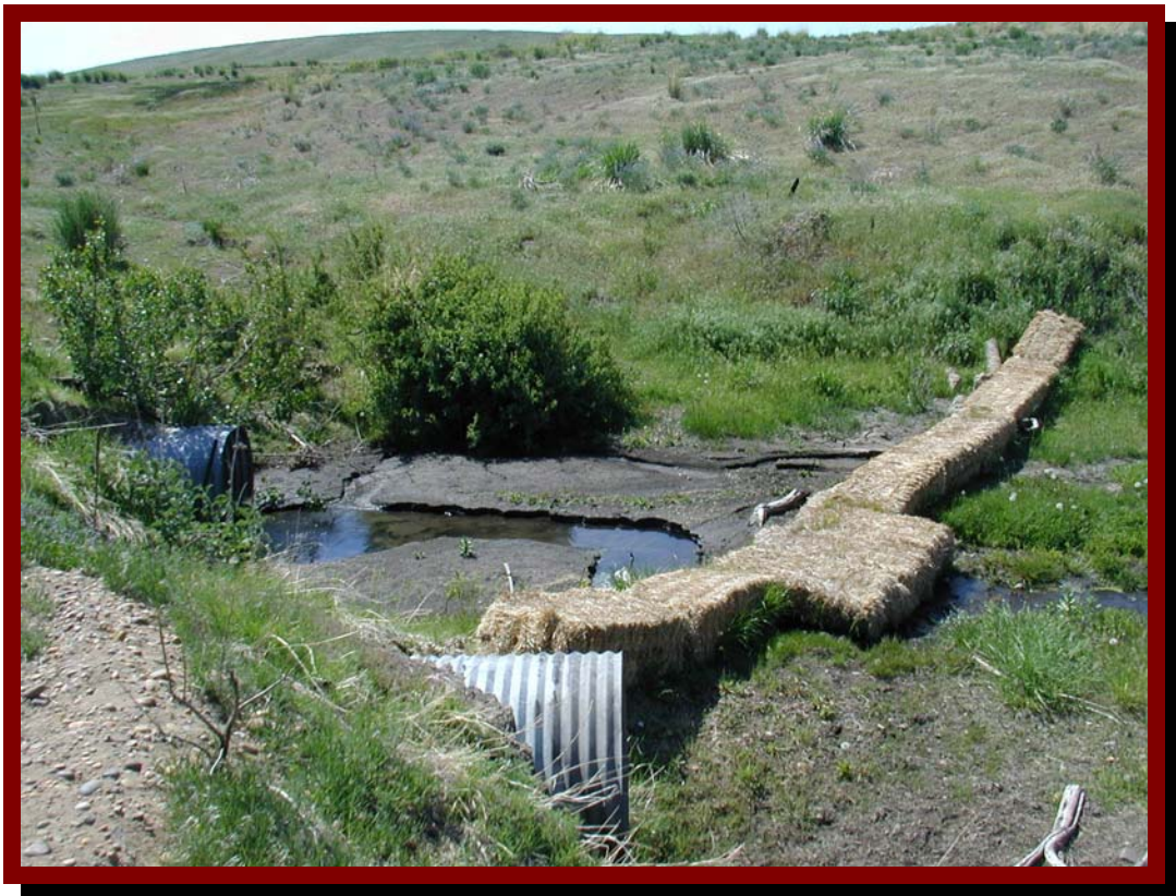
Figure 8. Sediment captured behind a bale structure on headwaters of Mule Creek.
