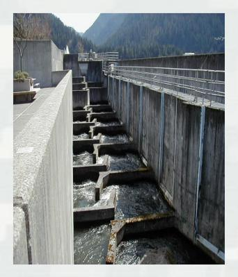
Vertical slot & orifice configuration
