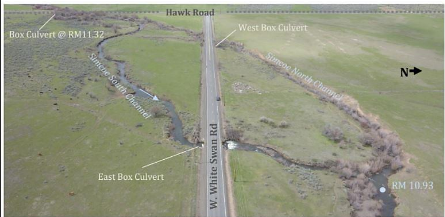
Figure 2. Simcoe South Channel Project Area. Photo (April 2019. IFI).
