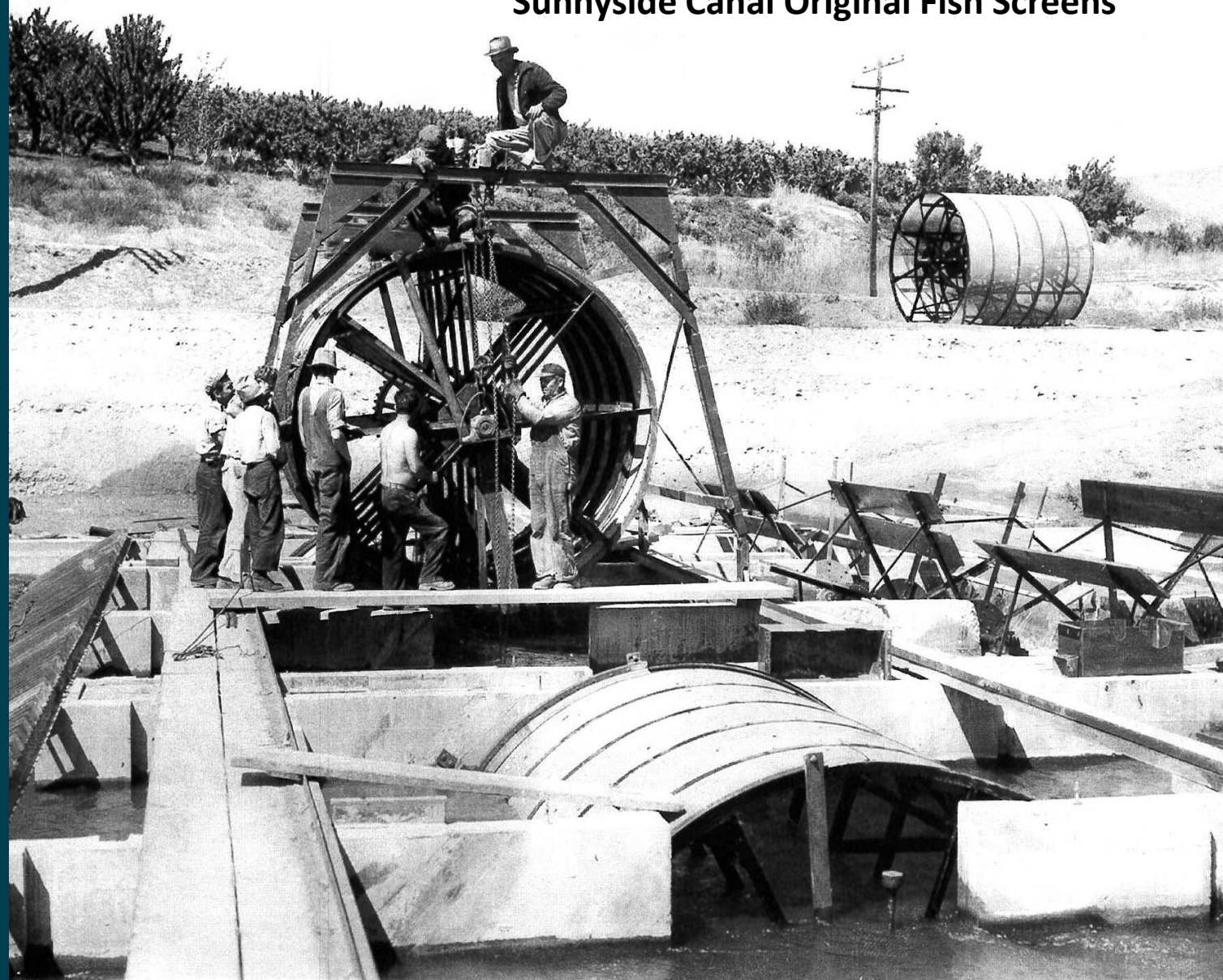
Sunnyside Canal Original Fish Screens
