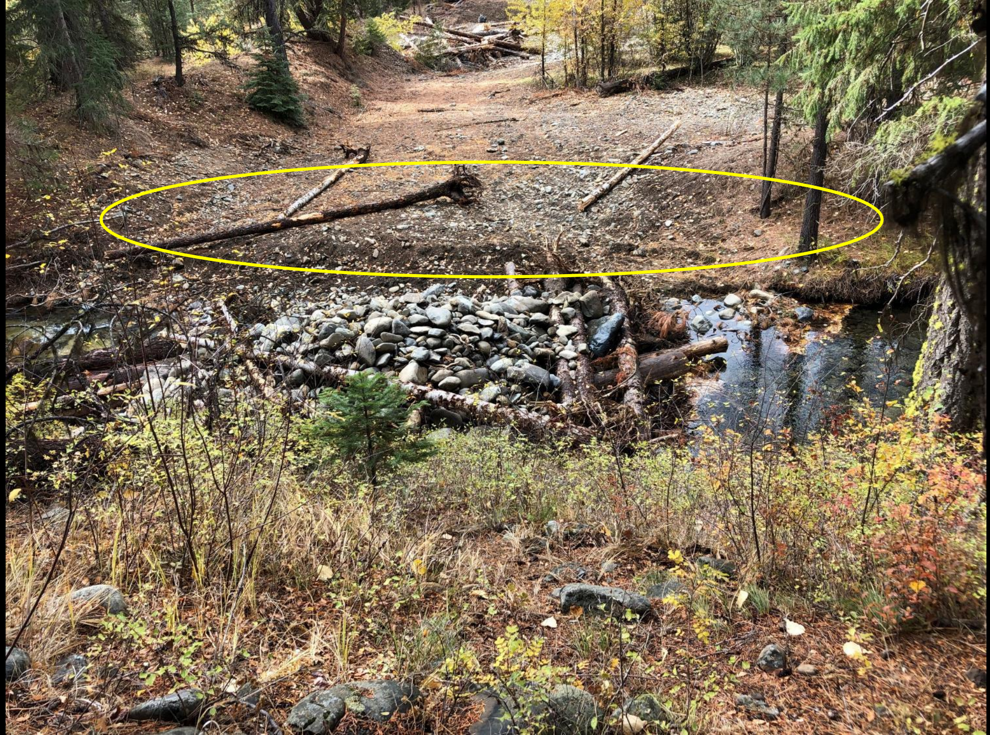
2021 wood structure and berm breach (circled)
