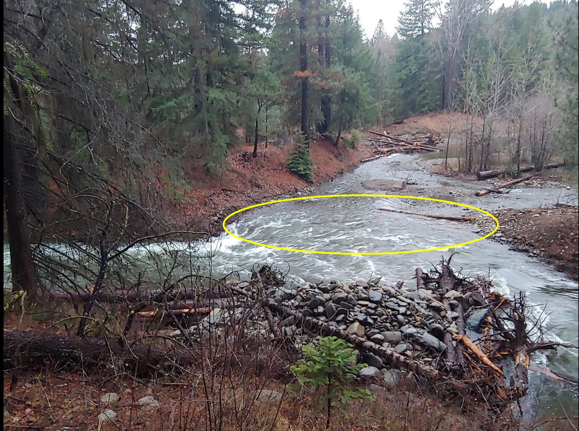
Wood structure directing flow into berm breach area, Nov. 13, 2021
