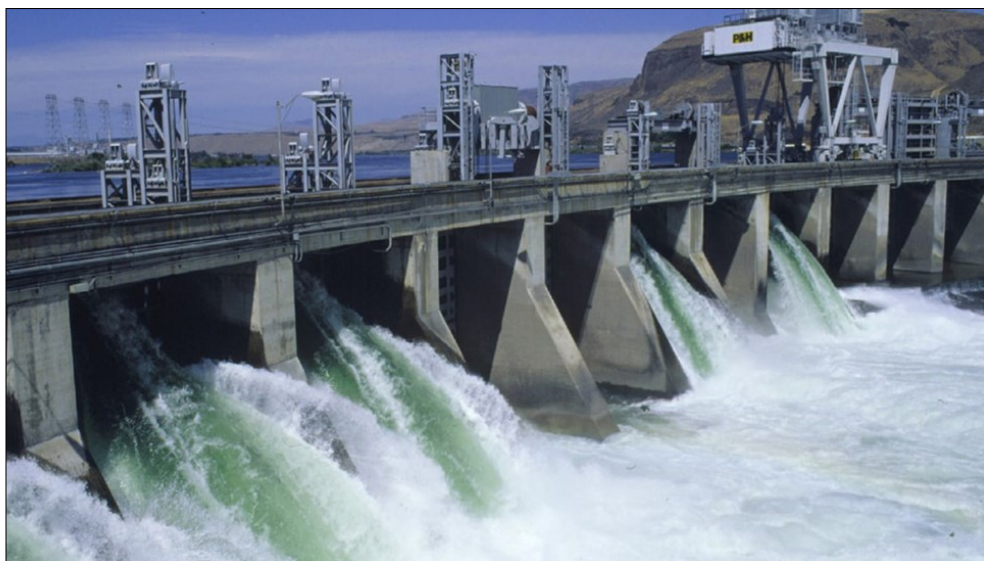
Above: Chelan County Public Utility's Rock Island Dam.
