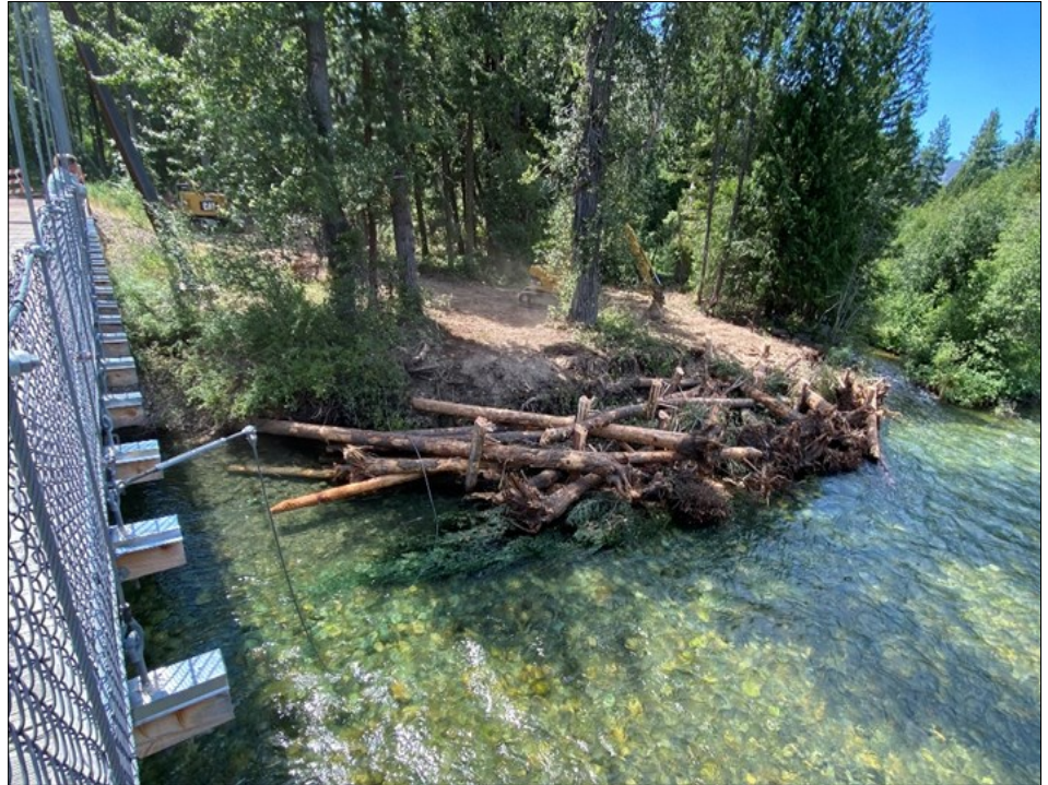
Above: Large wood structures upstream of the Suspension Bridge
