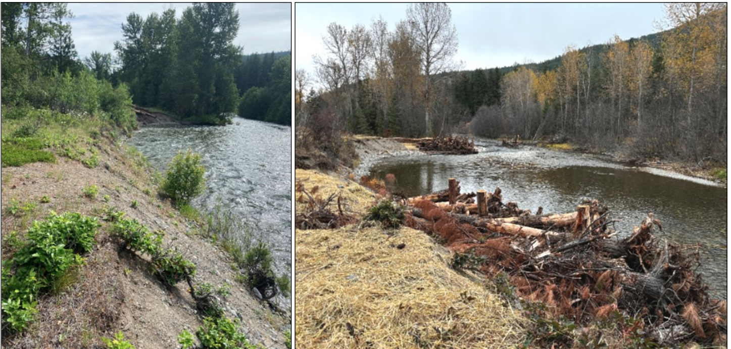
Above left: Project site pre-construction. Above right: Post-construction.
