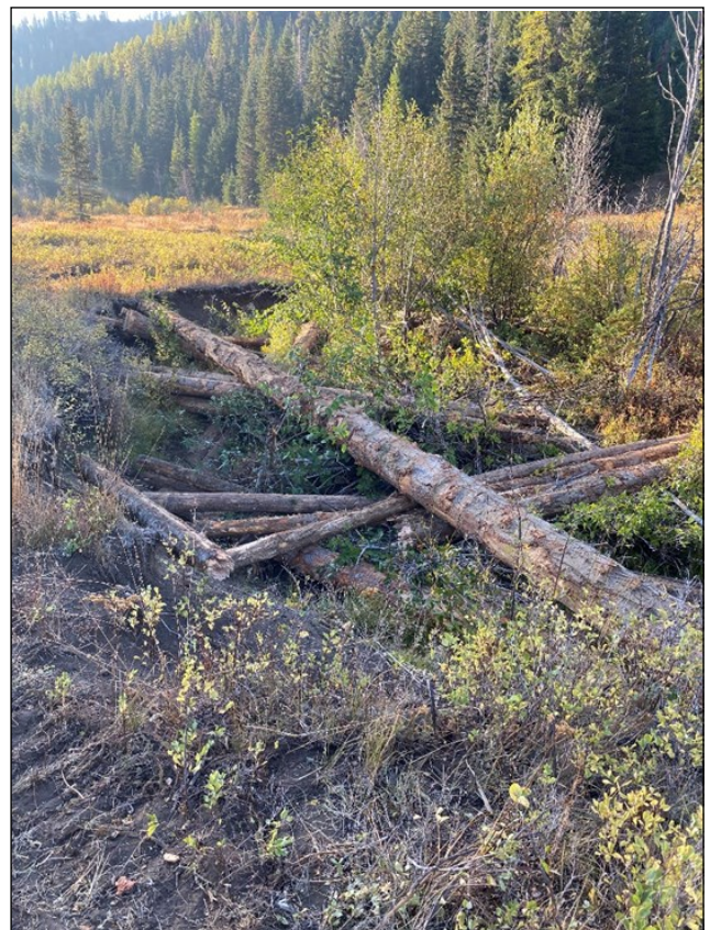
Above left: Example of channel incision and riparian degradation, NR Manastash Creek. Right: Ballast-based log jam after installation in stream channel.
