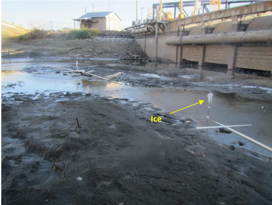
Figure 6. Overview of the PVC sprinkler system deployed downstream of the fish screens in the Sunnyside Canal in October, 2019, immediately after dewatering. Although ice accumulation (yellow arrow) was visible on the sprinkler shaft just below the spray nozzle, it did not prevent the sprinkler from operating properly. The same system was deployed in 2020 as well.
