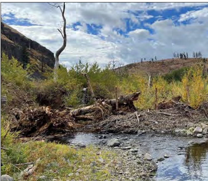
Wood structures installed in Swauk Creek included a channel spanning structure (left) designed to bolster existing beaver dams and a bar apex structure (right) that was keyed into the streambank. (YN)
