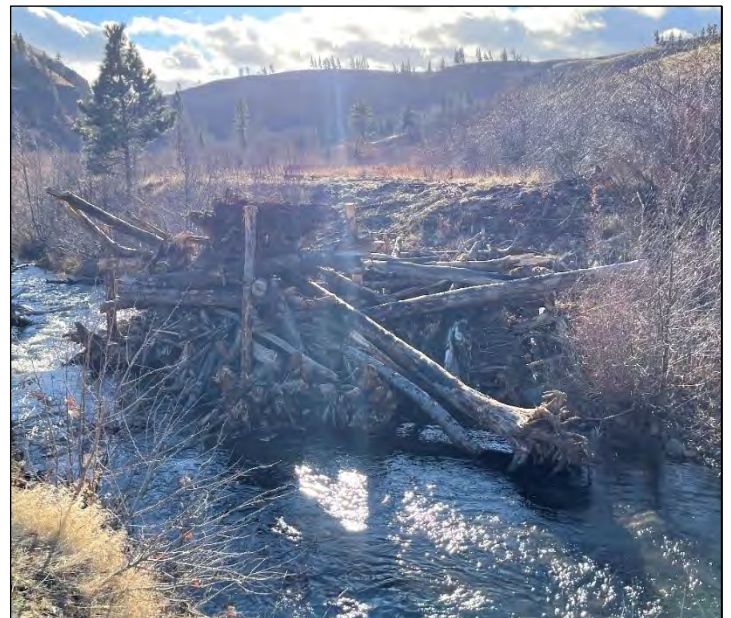
Wood structures installed in Swauk Creek included a channel spanning structure (left) designed to bolster existing beaver dams and a bar apex structure (right) that was keyed into the streambank. (YN)
