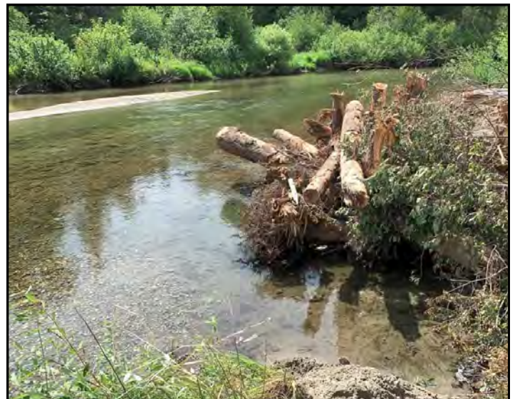
Side-channel habitat created and wood structures installed at the Nason Creek and the Wenatchee River confluence. (YN)
