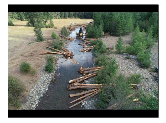
This example illustrates the magnitude of the wood replenishment in the stream channel. Notice the homogeneous nature of the existing stream channel. Increasing wood structure will help add some diversity to the channel.
