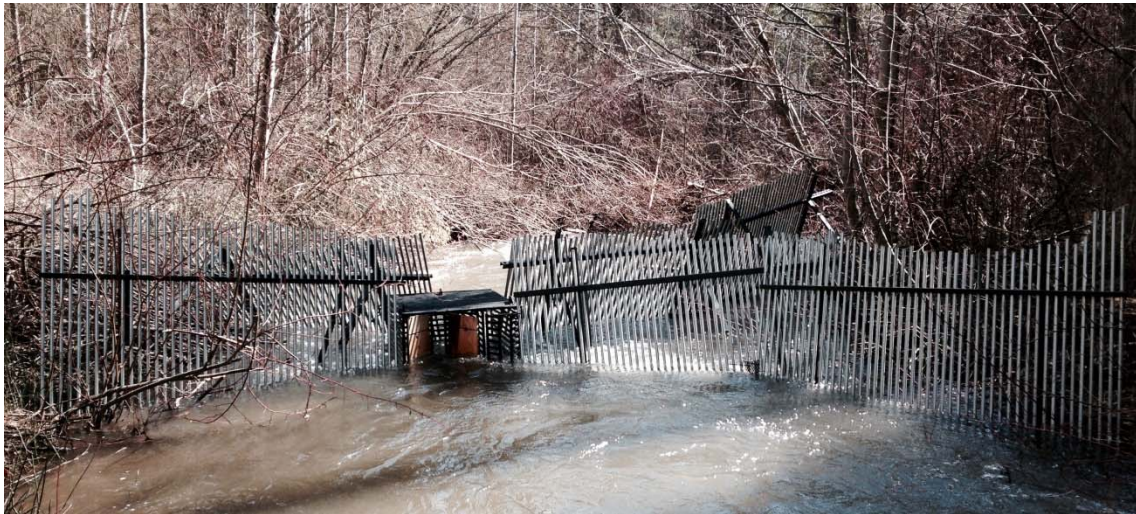
Figure 2.1 - Little Bridge Creek weir trap.
