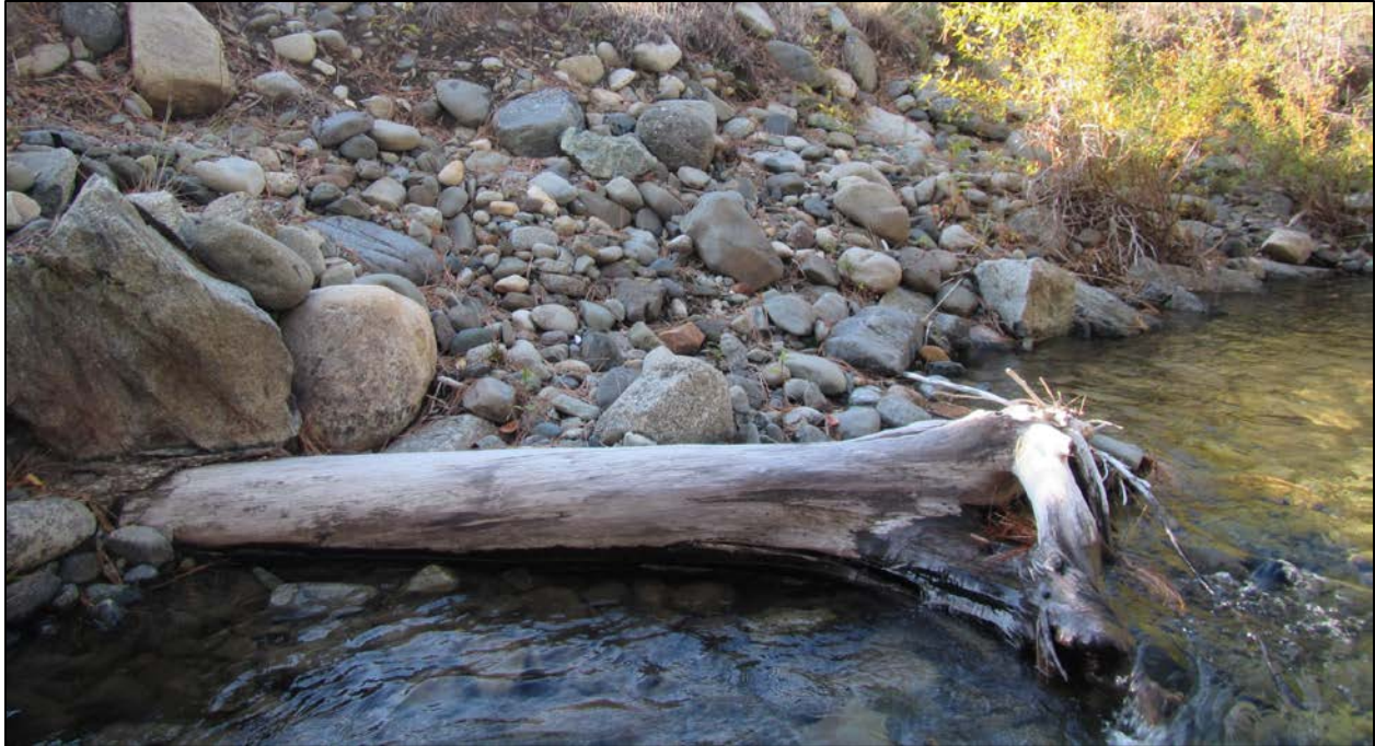
Figure 26. Partially buried LW at RM 0.05 on river right in Reach 1. (Photo: 10/1/19 )
