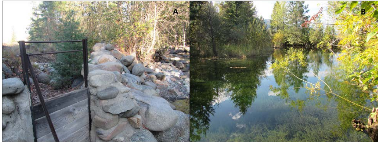
Figure 40. A) Boulder and cement irrigation outtake at RM 1.26 with leveed ditch in the background. B) irrigation-fed set of ponds on historical alluvial fan at RM 1 connected via ditches and culverts to the mainstem channel. (Photos: 10/1/2019)
