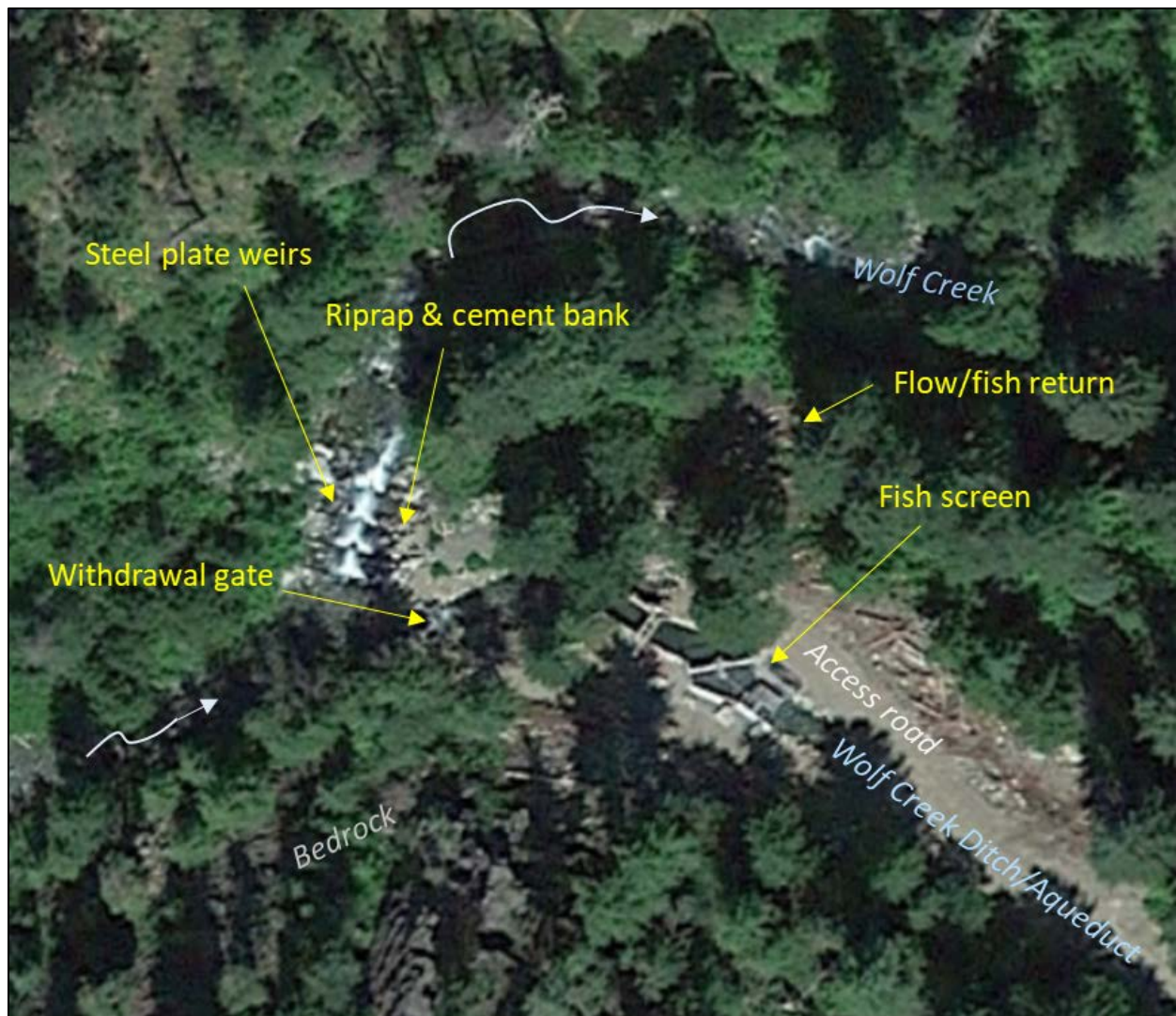
Figure 75. Overview of the Wolf Creek irrigation diversion at RM 4.53. (GoogleImage)
