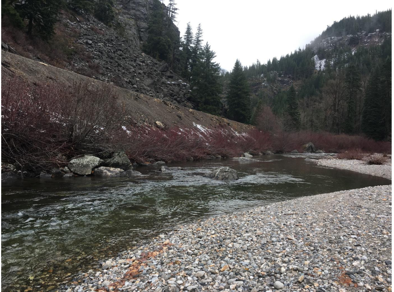
Figure 3. Railroad Grade Running Along Nason Creek Within the Upper Nason Reach.
