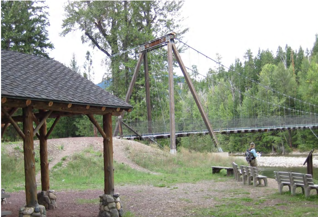
Figure 47. Suspension footbridge abutment and public area on downstream side of bridge on disconnected floodplain at RM 64.35. (9/3/2014)
