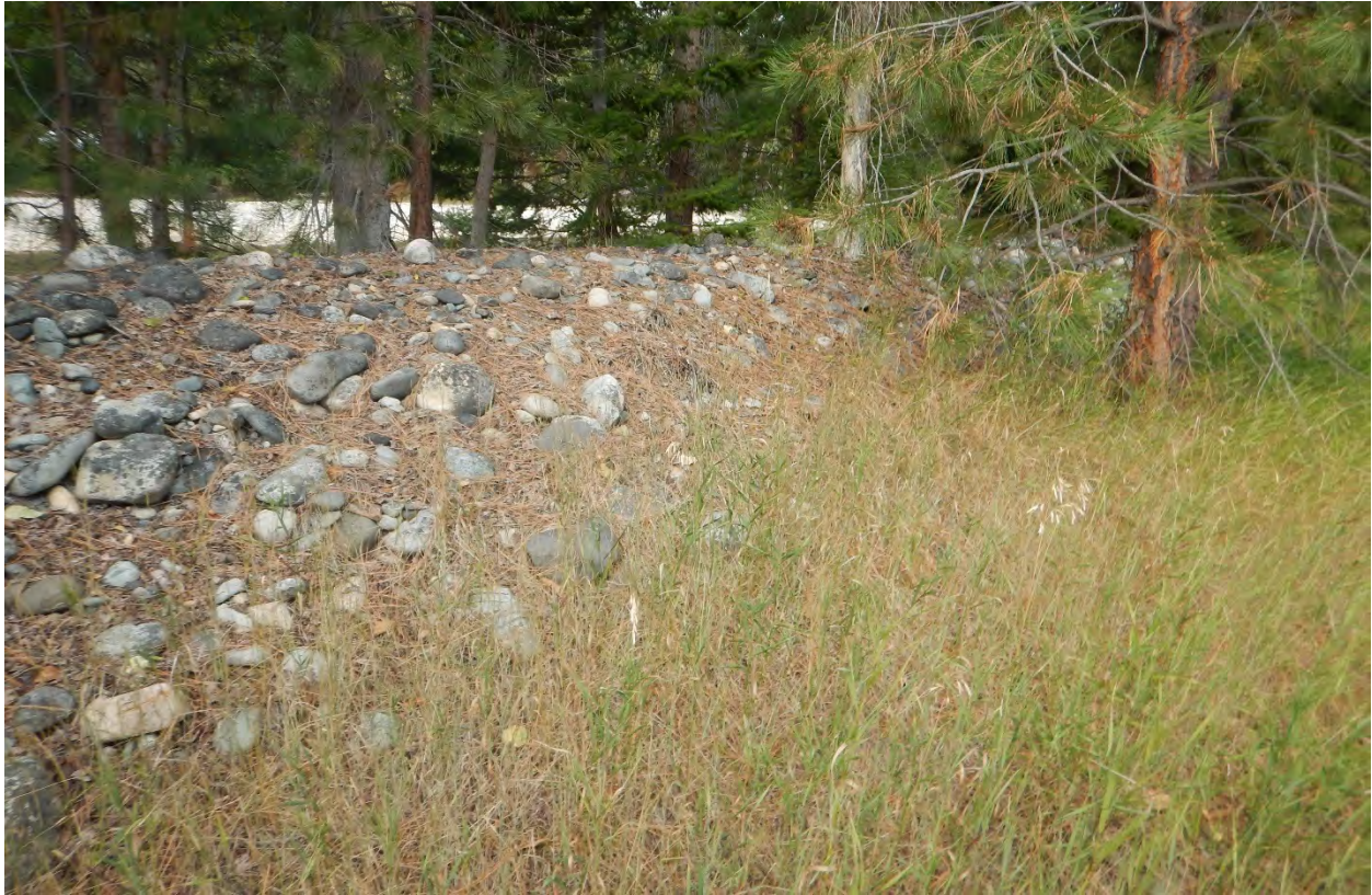
Figure 59. Push-up levee from land-ward side in Reach 3 on river-left at RM 65.35. (9/3/2014)
