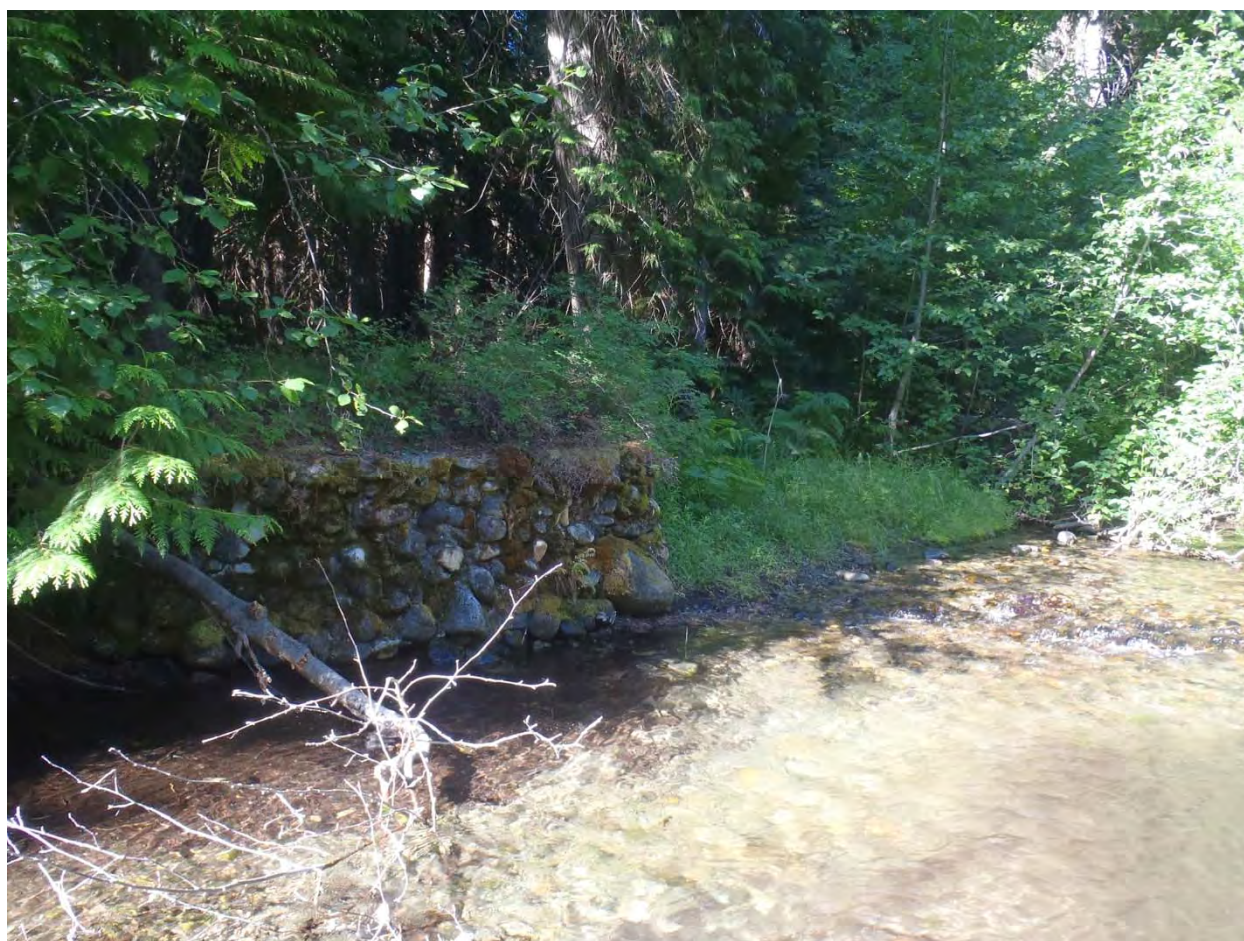
Figure 64. Remnants of an old bridge along SIDE25S.
