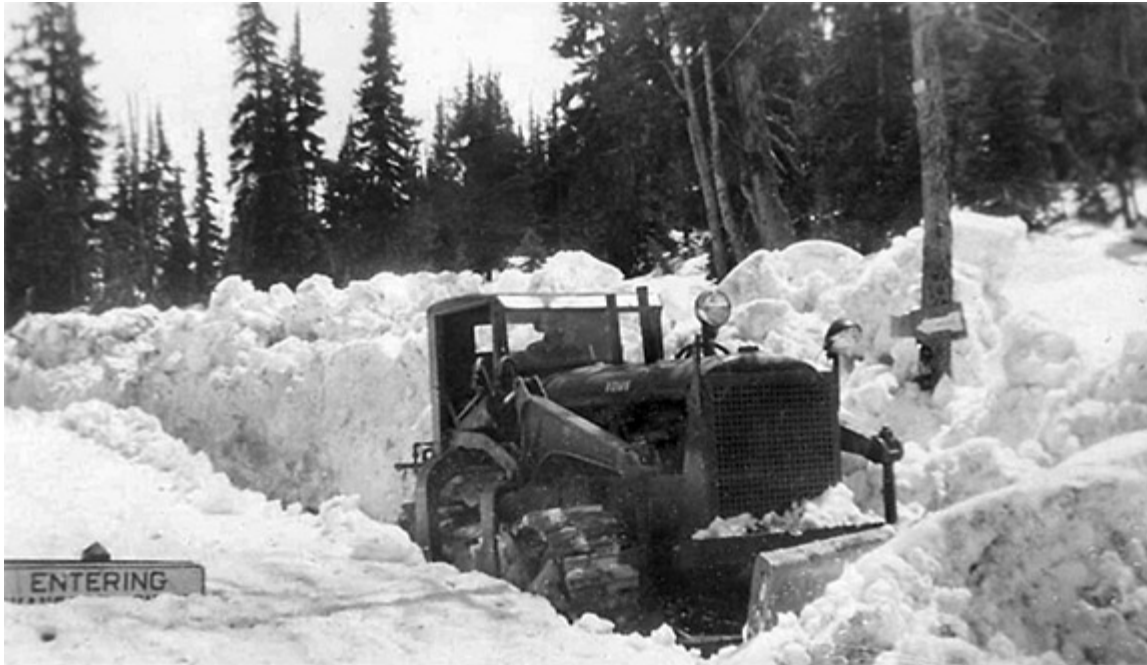
Figure 9. A tractor clearing deep snow along Hart's Pass. Date unknown, but probably during the war period of 1941-1945. Photo from the Frankie Waller Collection, courtesy of the Shafer Museum and the Methow Grist Archive.
