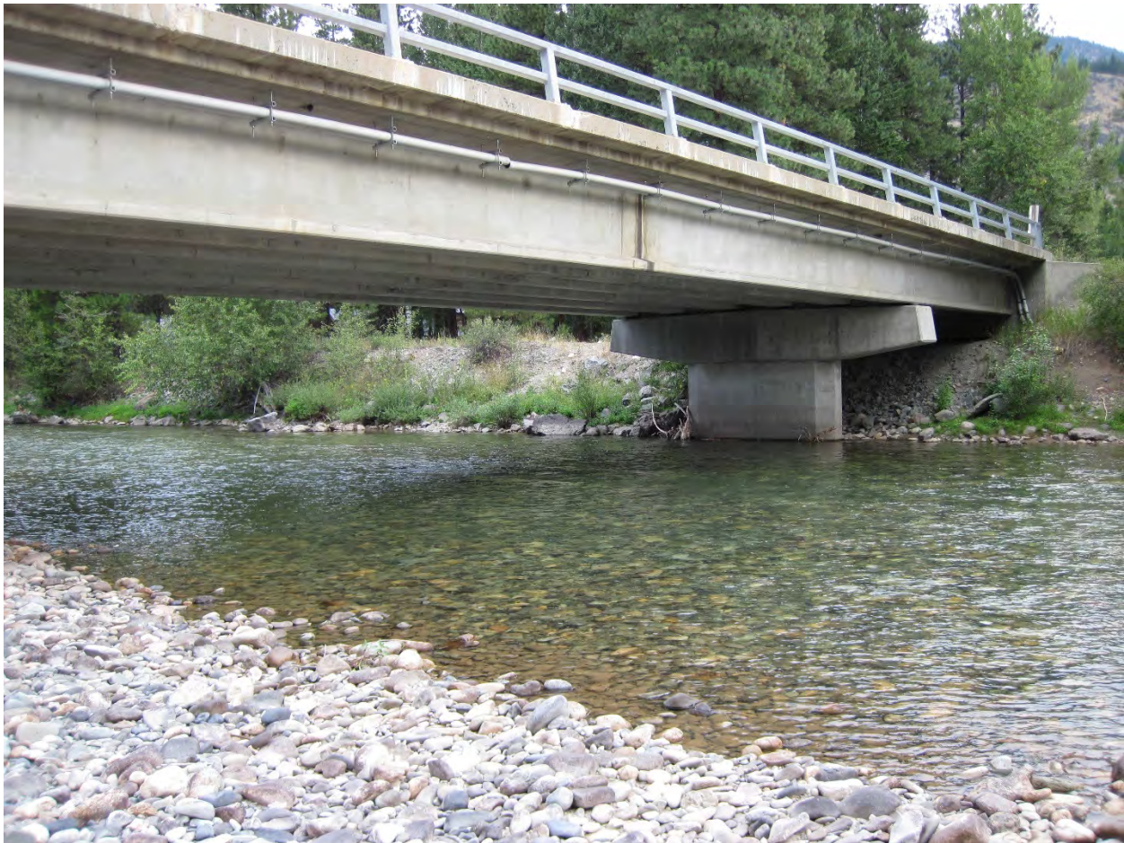
Figure 78. Mazama Bridge and riprapped bank on river-left (RM 67.2). (8/28/2014)
