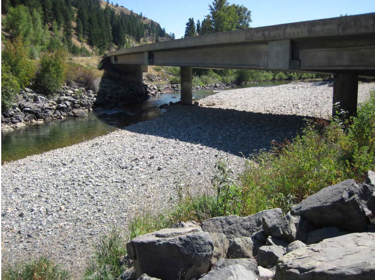
Figure 32. Weeman Bridge and the associated riprapped banks at RM 61.15. (9/5/2014)
