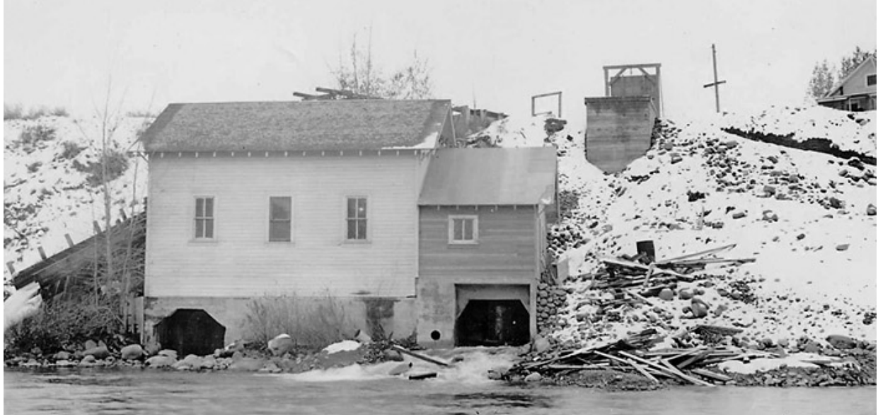
Figure 5. The first source of power for Winthrop came from diverted Methow River water that ran a generator, operated by the Upper Methow Valley Power and Light Company and located on the Methow River near the present-day East 20 Pizza. Photo courtesy Shafer Museum and the Methow Grist Archive.
