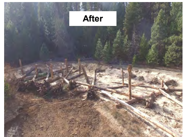
Floodplain reconnected and large wood installed (“after” photo taken before re-watering post-construction). (Photo: YN)
