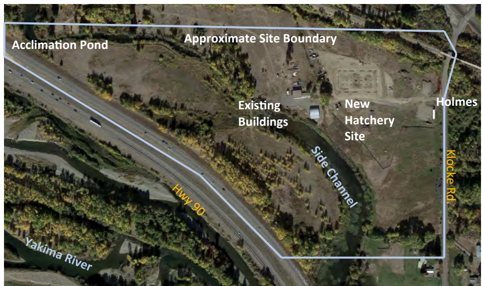
Aerial view of the hatchery site near Ellensburg WA during construction. (Photo: YN)
