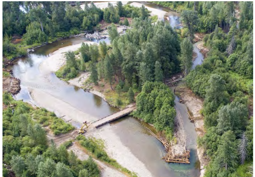
Project in progress, with temporary bridge in place. (Photo: YN)
