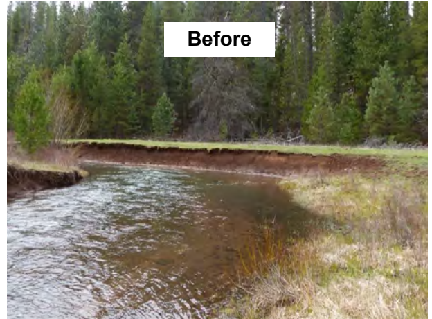
Stream disconnected from floodplain and downcut. (Photo: YN)
