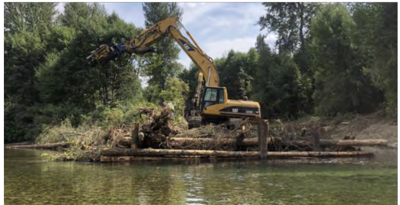
Log structure during construction. (Photo: YN)
