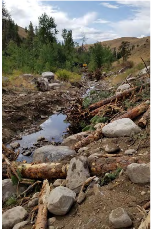
Completed new side channel. (Photo: YN)
