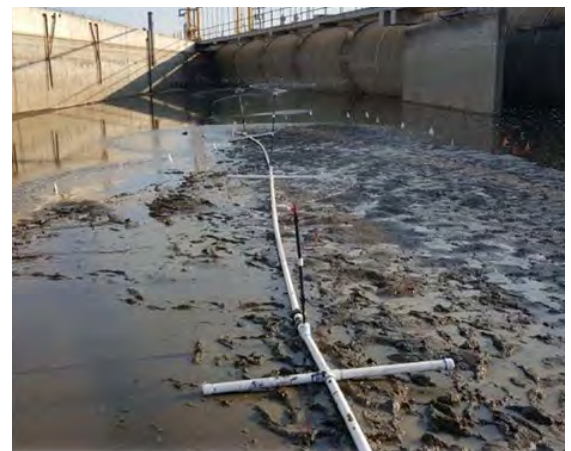
Sprinkler system used in dewatered irrigation diversions to keep juvenile lampreys wet. (Photo: YN)
