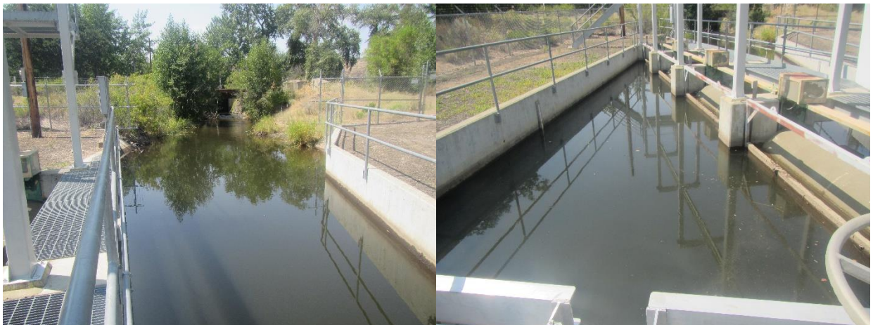
Figure 8. Overview of above the drum screens (right) and an overview of below the drum screens (left) at the Upper WIP Diversion on Ahtanum Creek, taken July 31, 2018.
