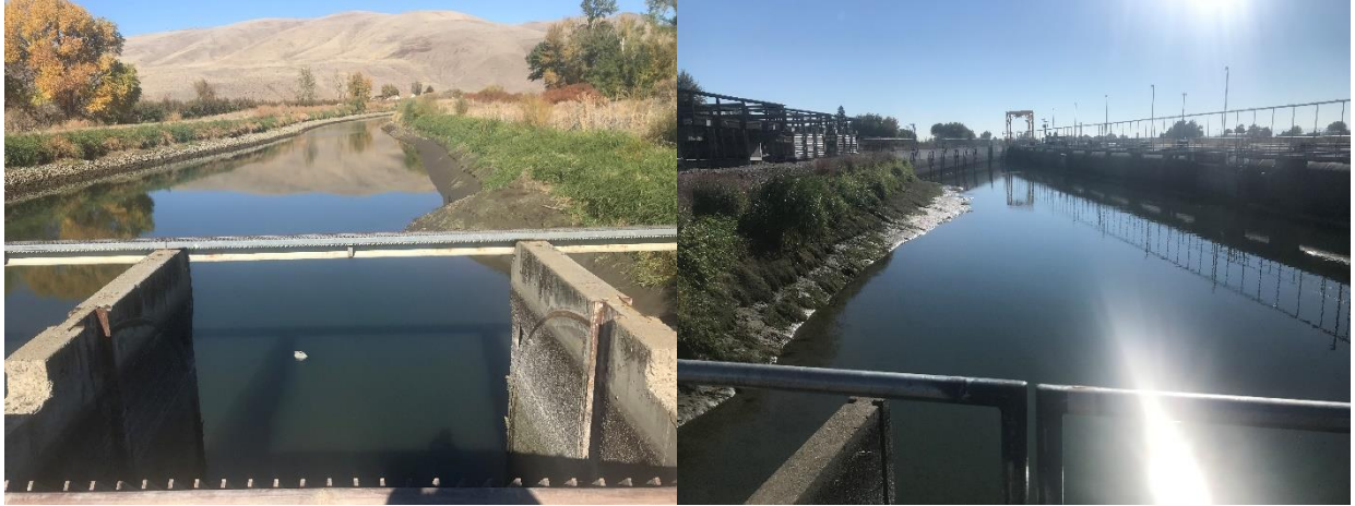
Figure 3. Overview of the upstream area above the trash racks (right) and the upstream area below the trash racks (left) taken October 17, 2018.
