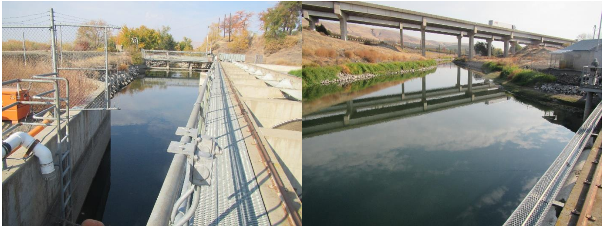
Figure 1. Overview of downstream area of the drum screens (right), and upstream of the drum screens (left) before dewatering at Sunnyside diversion on October 23, 2018.
