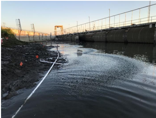
Figure 4. Overview of Sprinkler system setup, taken October 17, 2018.
