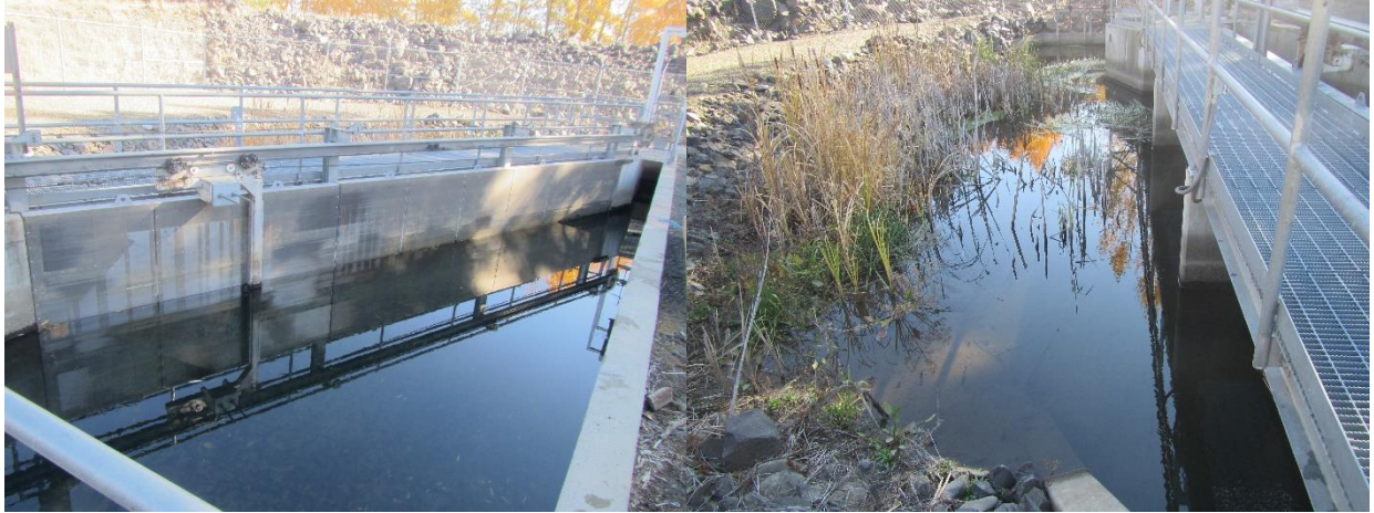
Figure 14. Overview of above the screens, below the trash racks (right) and overview of below the screens at the Ellensburg Mill Diversion on the Yakima River before dewatering, taken October 23, 2018.
