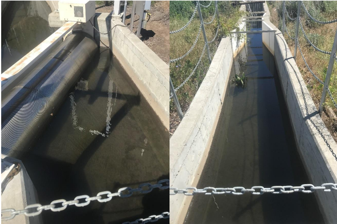
Figure 5. Overview of above the drum screen directly by the screen (right) and the upstream section that tapers into the canal (left) from Diversion 14 on Ahtanum Creek, taken on July 3, 2018.
