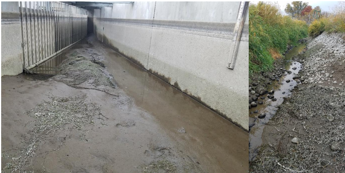
Figure 15. Overview of below the screens (right) and looking down the canal (left) of the New Cascade Diversion on the Yakima River, taken on October 23, 2018.
