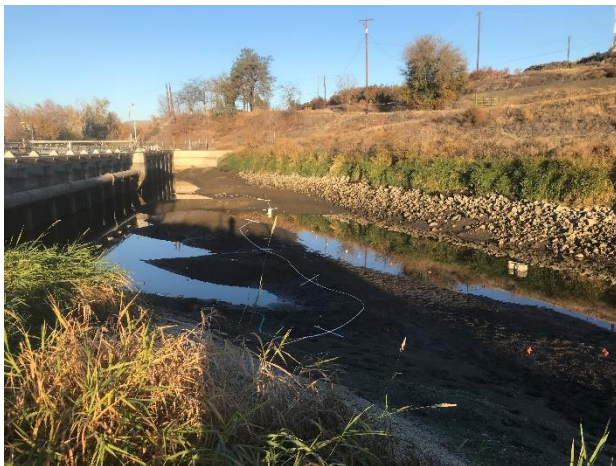
Figure 2. Overview of downstream area of the drum screens after dewatering at Sunnyside diversion on November 8, 2018.
