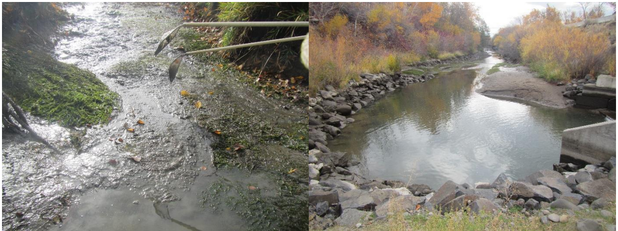
Figure 10. Close up of sampling area above the screens (right) and overview just below the head gate looking down the canal at Wapatox Diversion on the Naches River, take November 1, 2018.
