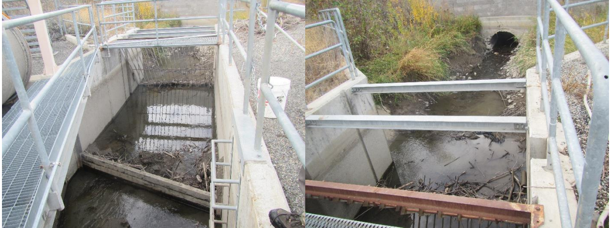
Figure 9. Overview of above the screens, below the trash racks (right) and an overview of above the screens, above the trash racks of the City of Yakima Diversion on the Naches River, taken November 1, 2018.
