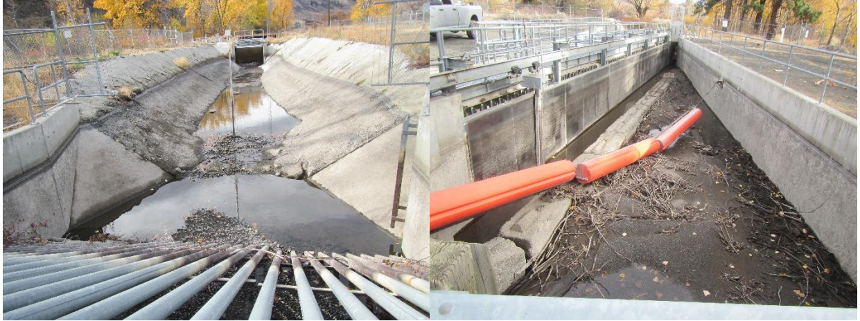
Figure 11. Overview of above the screens, above the trash racks (right) and overview of the dried sediment and isolated pools above the screens, below the trash racks (left) of the Naches-Selah Diversion on the Naches River, taken November 1, 2018.
