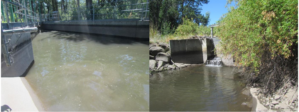
Figure 7. Overview of above the drum screens (right) and the closed headgate that feeds the canal (left) at the Bachelor-Hatton Diversion on Ahtanum Creek, taken July 19, 2018.
