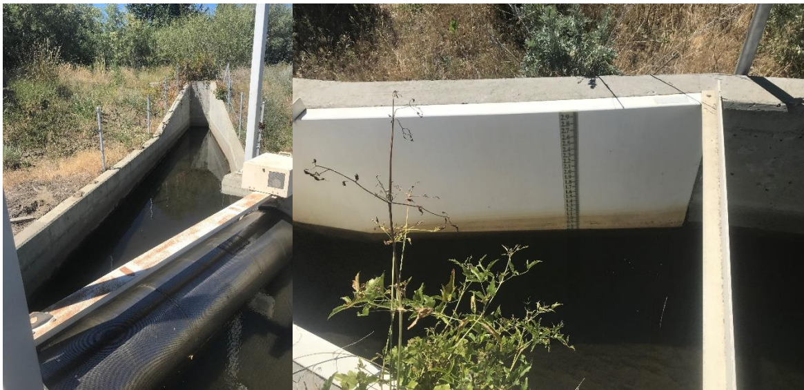
Figure 6. Overview of below the drum screen (right) and the water gauge (left) from Diversion 14 on Ahtanum Creek, taken July 3, 2018.
