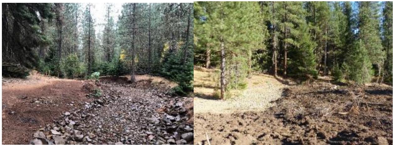
Figure 6. Channel conditions after Type 2 rock fill (left) and post de-compaction (right).
