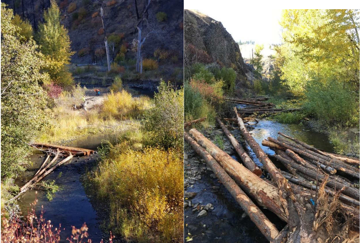
Figures 6 & 7. Photos of wood placement post implementation.
