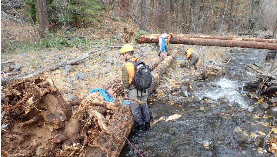
Figure 6. Photo of biologists directing placement of wood in Little Rattlesnake Creek during implementation.
