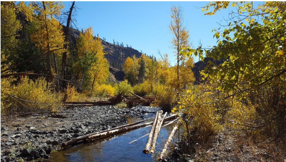
Figure 8. Photo of wood placement post implementation.
