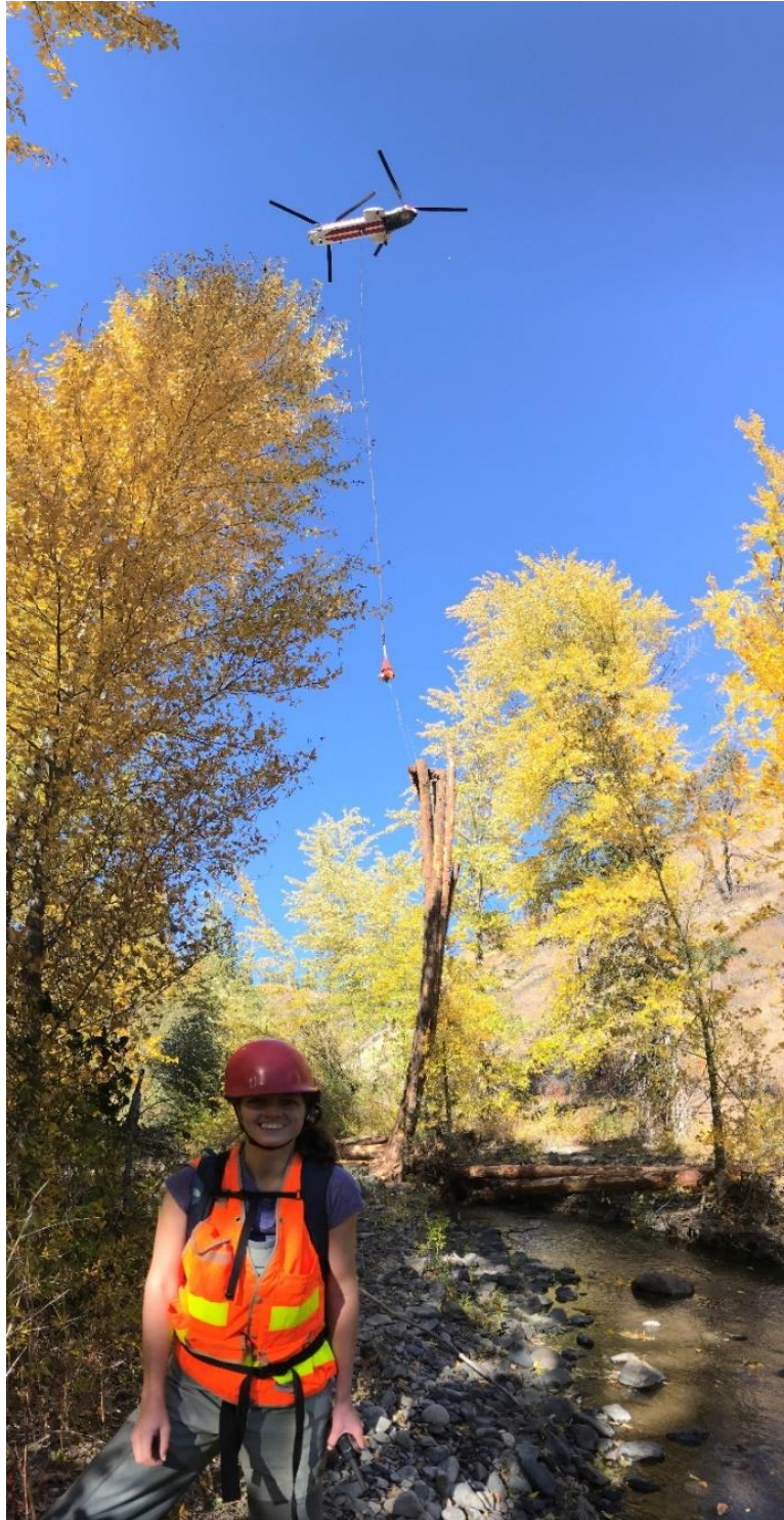
Figure 5. Photo of the 107-Vertol helicopter placing wood instream during project implementation.
