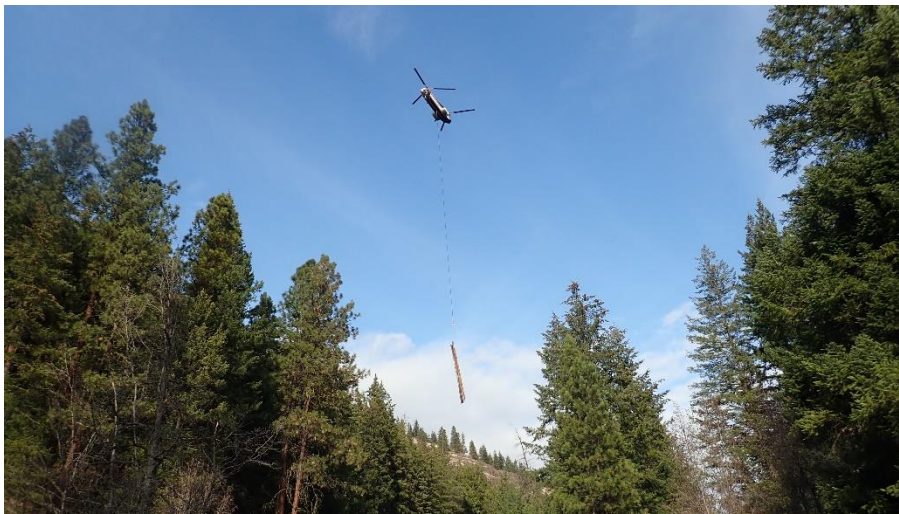
Figure 5. Photo of helicopter during implementation flying logs into Little Rattlesnake Creek.
