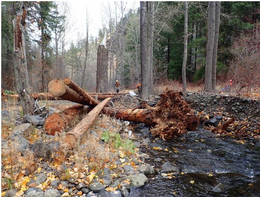
Figure 7. Photo of wood placement in Little Rattlesnake Creek.
