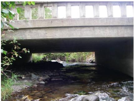
Figure 12. Habitat alteration and channel confinement at the Hwy 153 Bridge (RM 0.3).
