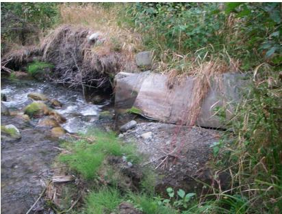
Figure 35. Plywood armoring along river-right near the downstream end of Reach 2 (September 2011).
