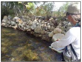
Figure 6. Riprap wall near RM 0.11. The top elevation is approximately 5.5 ft above OWH.
