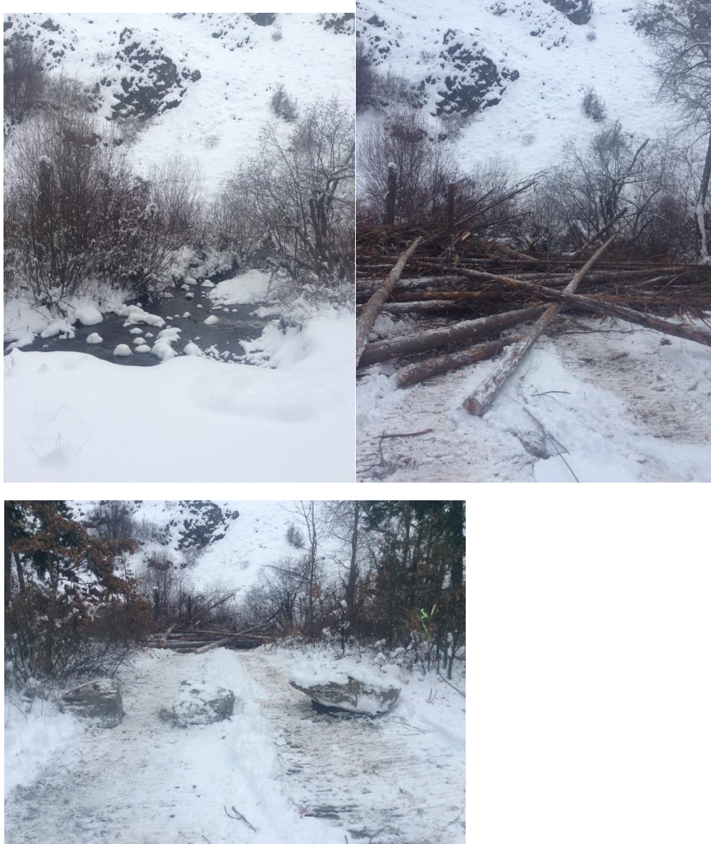
Figure 5 – Site 2 before and after wood placement. Boulders place to exclude vehicular access December 2016.
