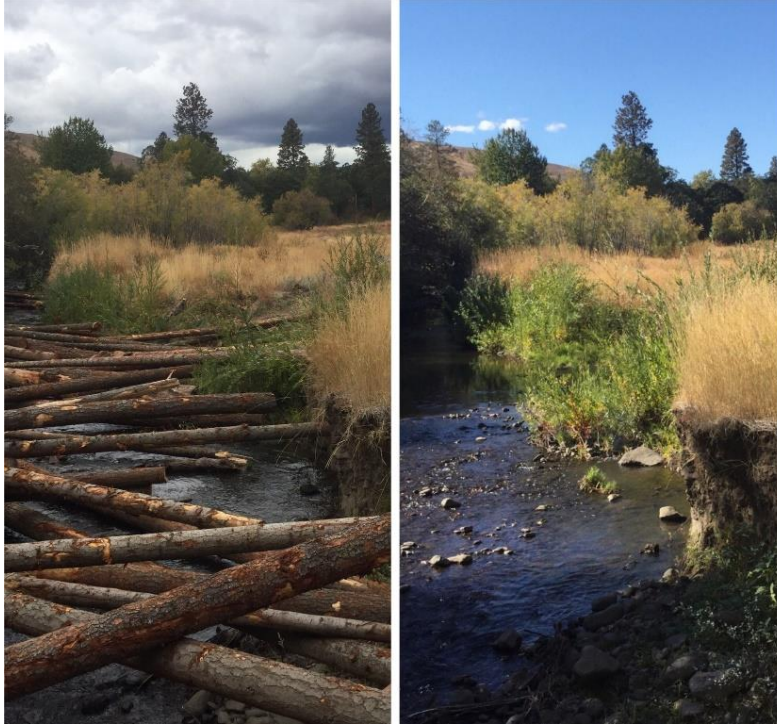
Figure 4. Before (October 3, 2016) and after (October 6, 2016) photos of wood placement at site #1
