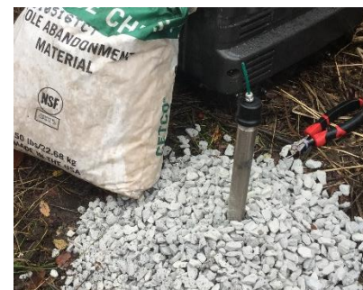
Figure 8. Bentonite clay to stabilize well
