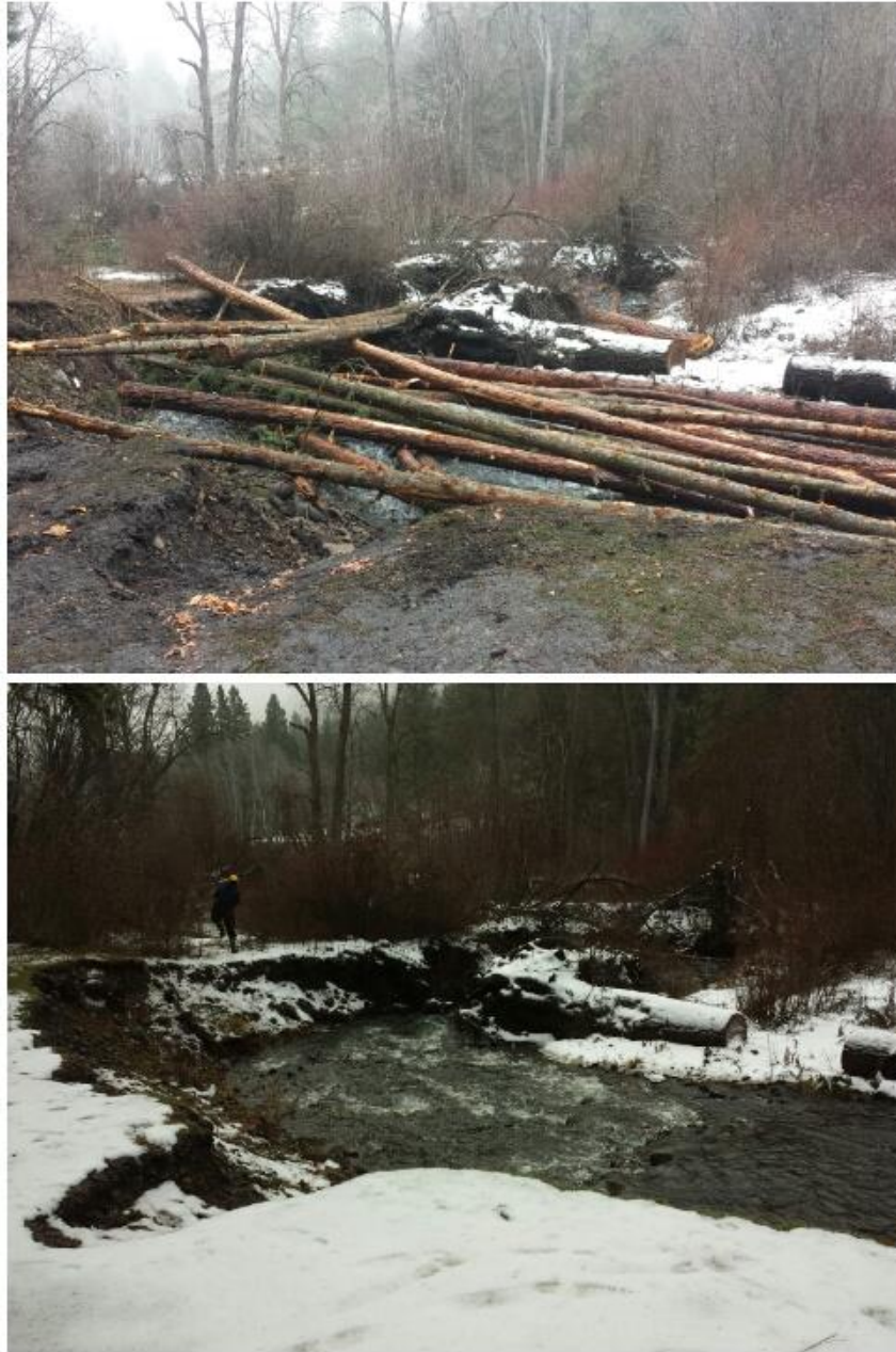
Figure 2. Before and after construction
