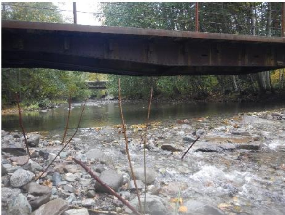
Figure 1. Before and after construction
