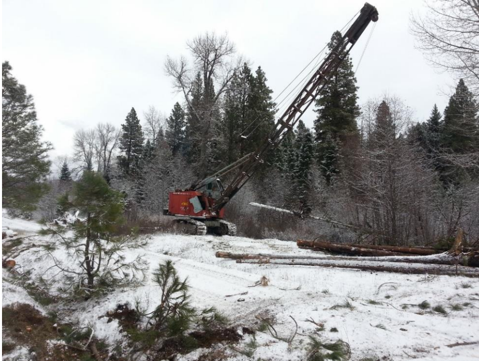
Figure 14 Indian Creek Floodplain during restoration.
