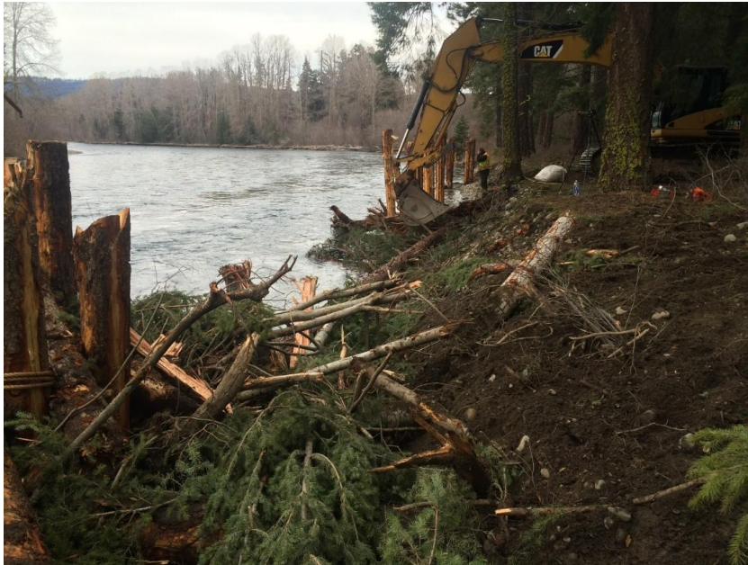
Figure 10 Habitat conditions during Type 1 log jam construction
