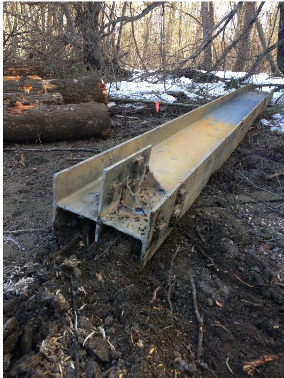
Figure 8 Modified H-Pile used to produce a bore for wooden pile driving
