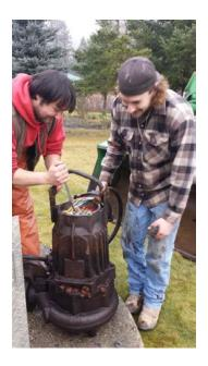
Raincountry Refrigeration removing one of the two recycling sump pumps. The pump was removed in January 2015 and a rebuilt one will be installed after the June 30, 2015 time period. Future work wil include the replacement of both pumps as they have accumulated over 95,000 hours of operation.
