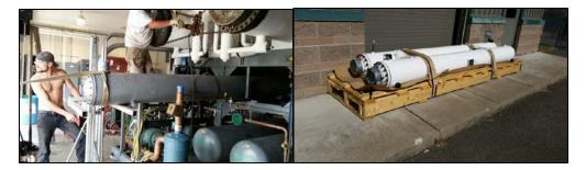
Two photos above, one showing removal of old condenser and the other on the right show the two replacment condensers that will be plumbed and ready for the 2015 egg incubation period.
