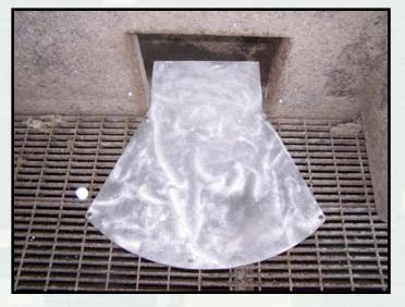
Diffuser plating at weir orifices
