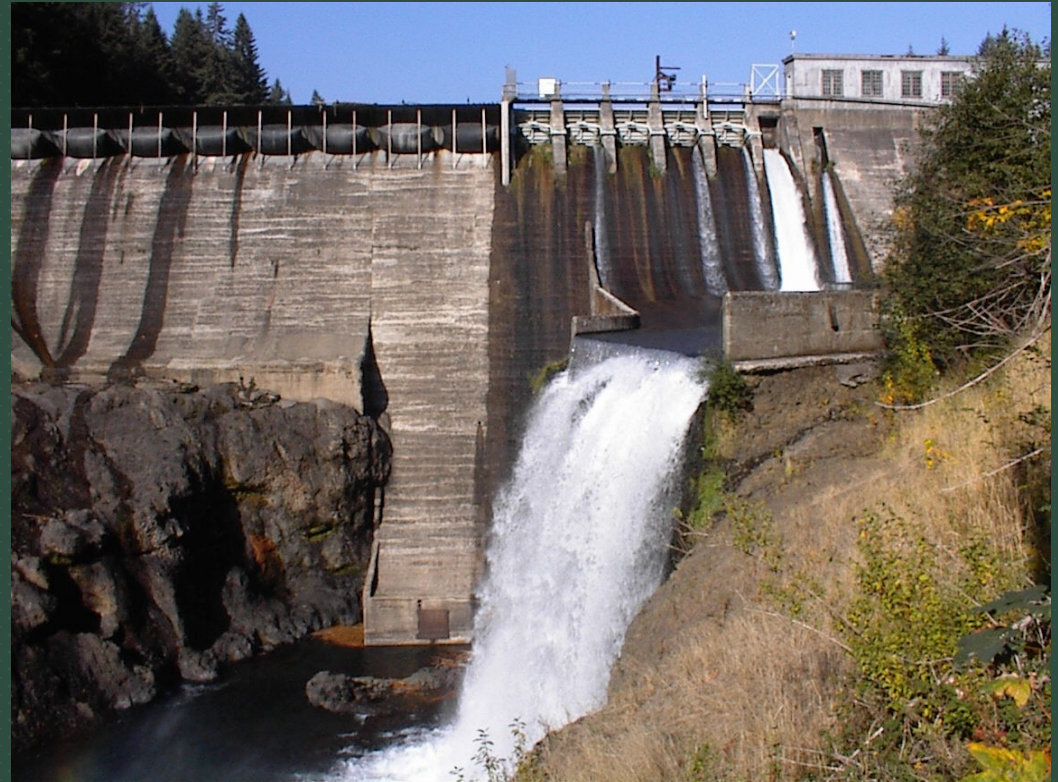
Condit Dam, White Salmon River Basin (WA)
