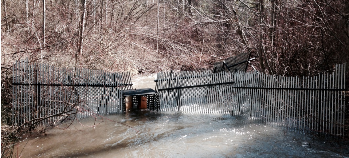
Figure 2.1 - Little Bridge Creek weir trap.
