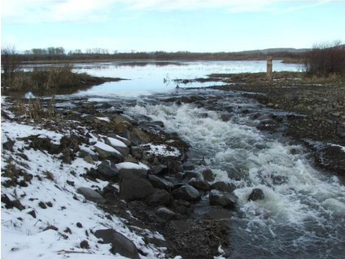
Figure 3. Rebuilt spillway out of Circle Lake in December 2015, Satus Wildlife Area.
