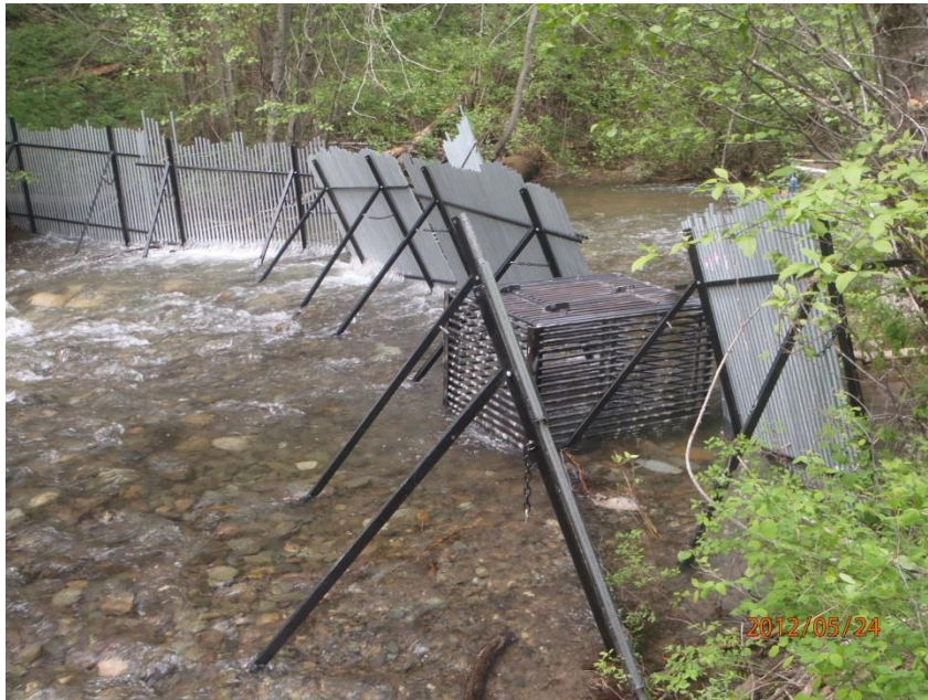
Figure 2.1 - Little Bridge Creek weir trap layout and trapbox from downstream
