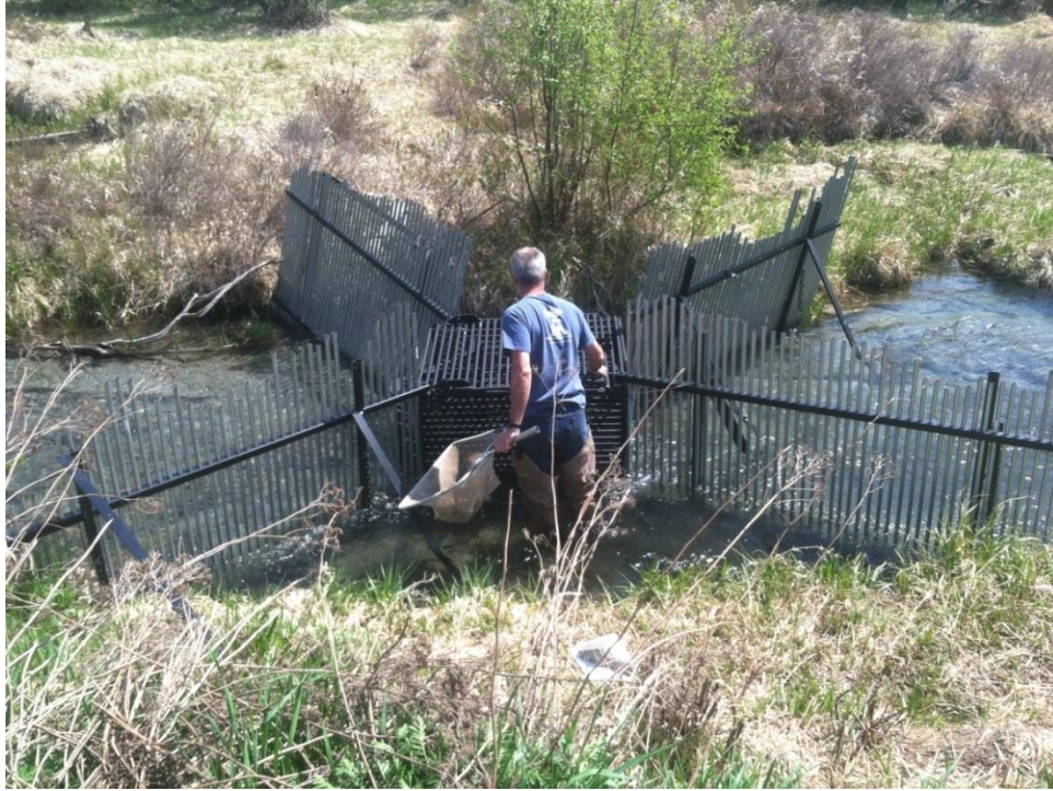
Figure 2.3 - Hancock Springs weir
