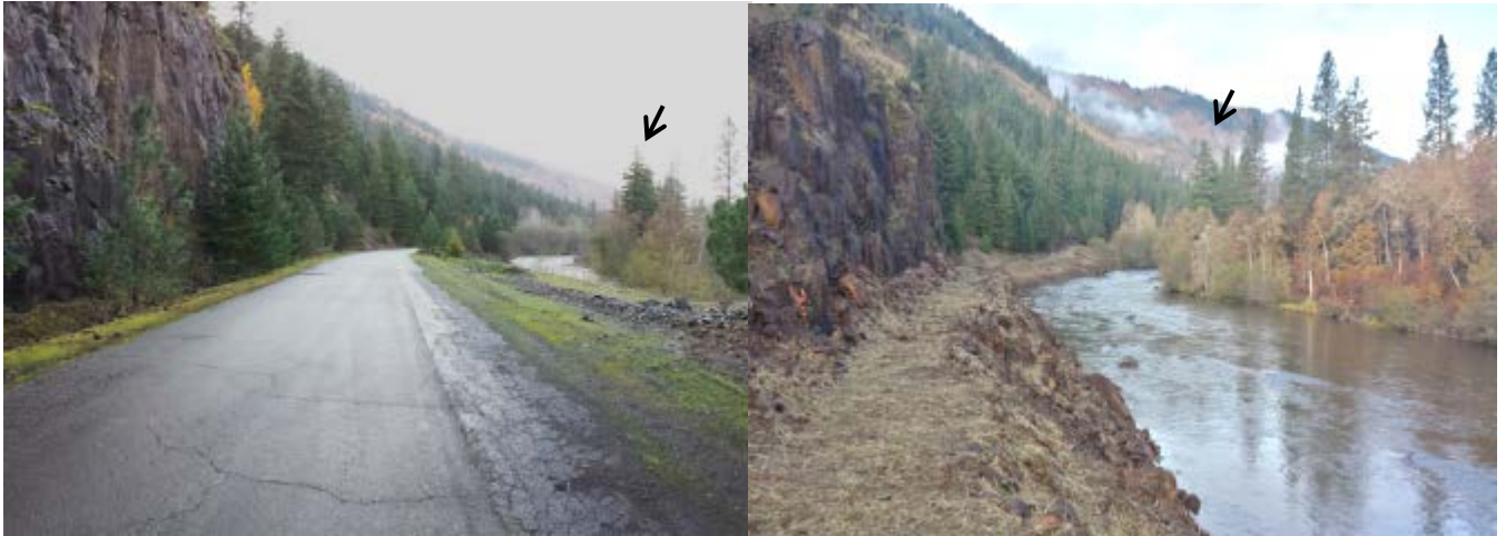
Figure 10. Example of daylighting of bedrock feature, pre- (left) and post-project (right).
