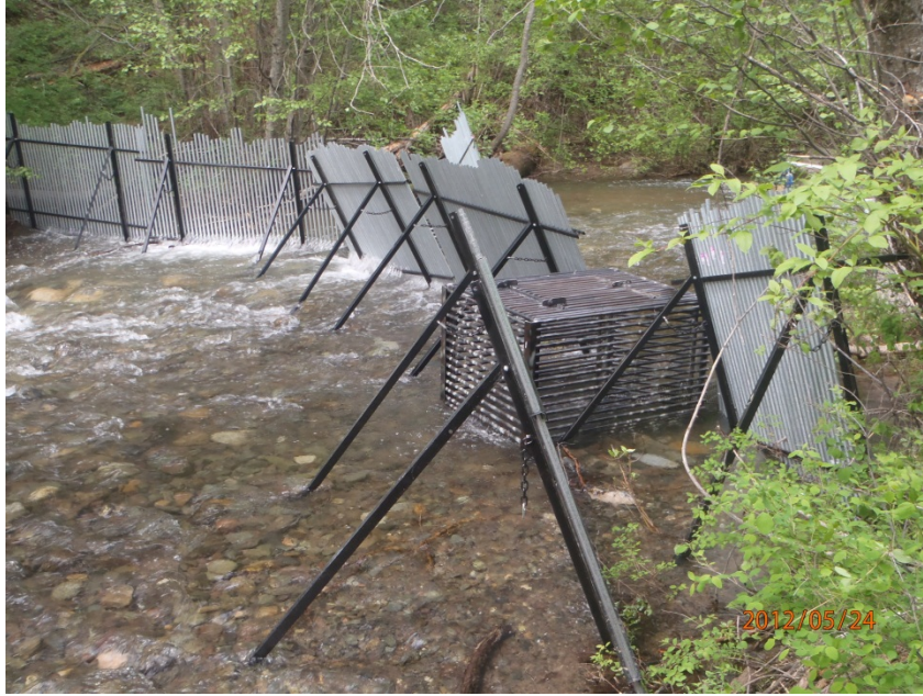
Figure 2.1 - Little Bridge Creek weir trap layout, downstream view.
