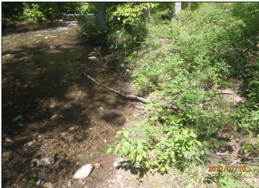
Figure 0.4 - Road Approach: Post-Installation
