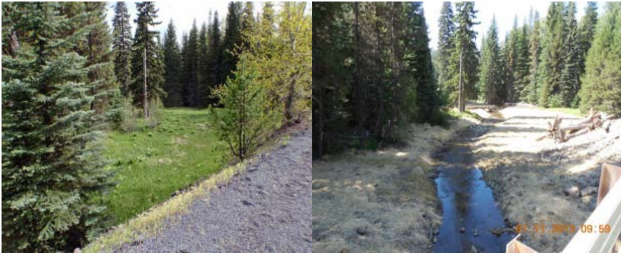
Figure 4. Upper Klickitat River In-channel and Floodplain Enhancement – Phase 3 pre (left) and post bridge installation (right) looking in the downstream direction below the 255 rd-xing.
