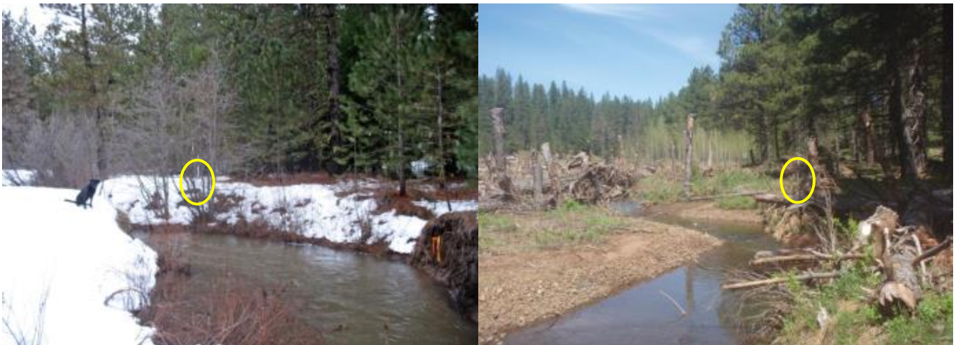
Figure 8. Tepee Creek Meadows Restoration – Phase 2 pre (left) and post riffle construction (right) and LWD placement, well (yellow circle) placement is consistent in both pictures although “post” picture is taken with a wider angle.
