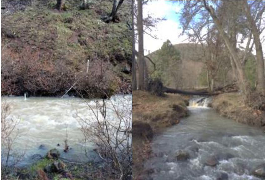
Figure 13. New streamflow gaging stations installed in 2012, Wheeler Creek (left) and Logging Camp Creek(right).
