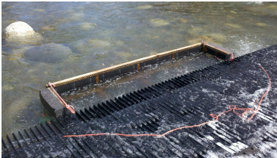
Figure 4.5 - Modified trap installed at Twisp Weir.
