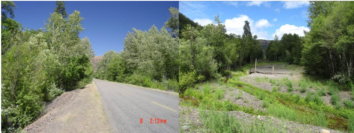
Figure 15. Before (left) and after (right) removal of road prism, construction of channel, and grading of floodplain (Phase 2).
