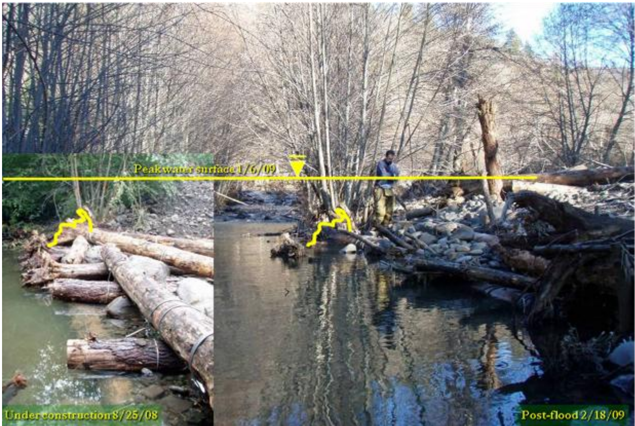
Figure 19. Element 4 during construction (inset) and post-flood.
