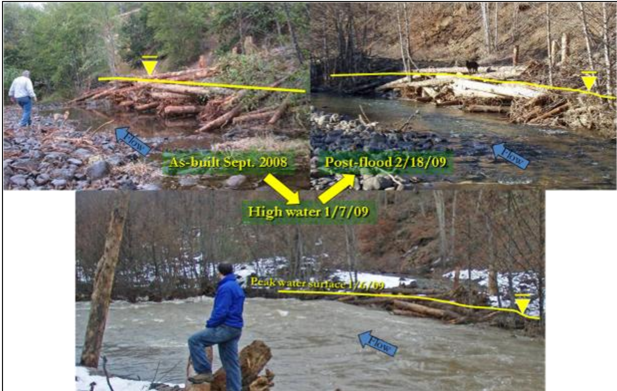
Figure 20. Element 5 as-built (top, left), during flood (bottom), and post-flood (top, right).
