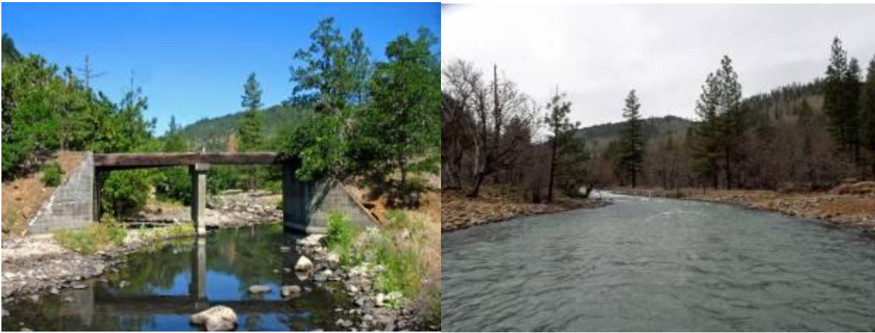
Figure 17. Upstream view of railroad crossing before (left) and after (right) treatment.
