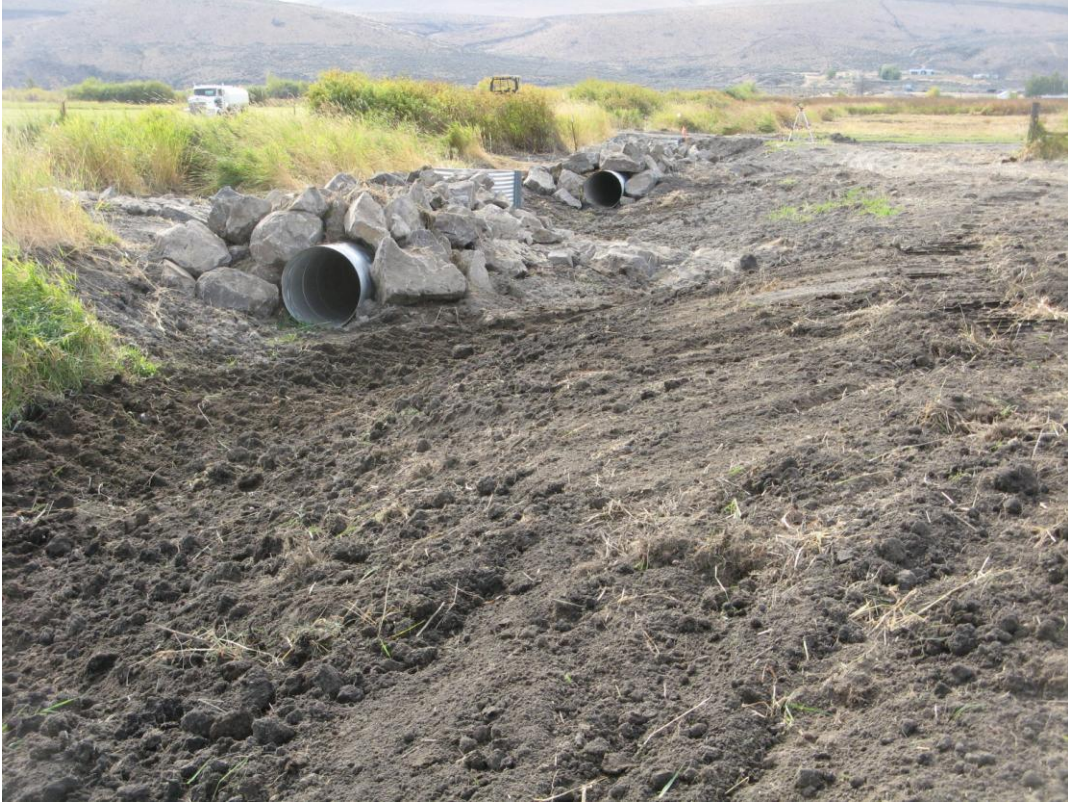
Water Control Structures soon after installation
