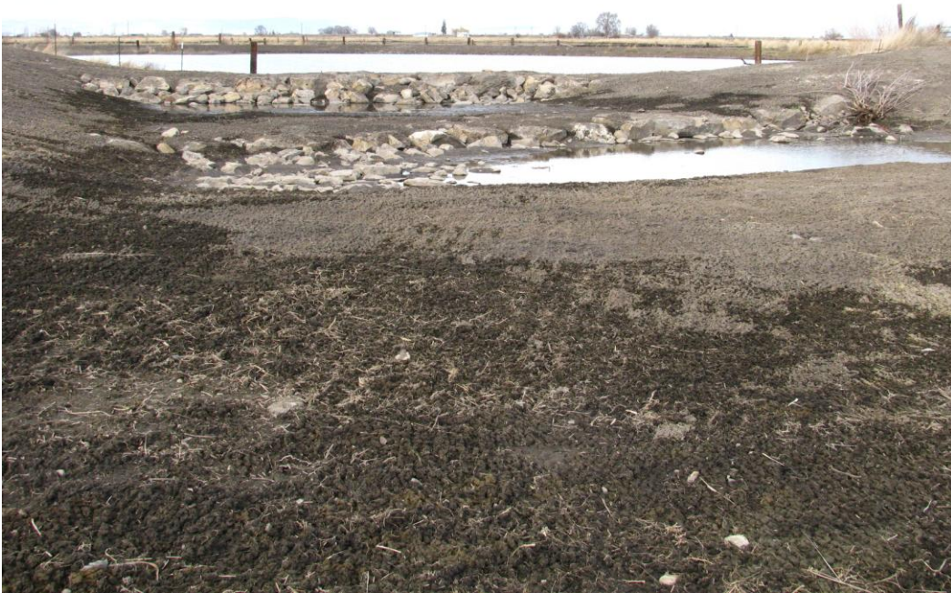
Spillways at lower portion of restored wetland.
