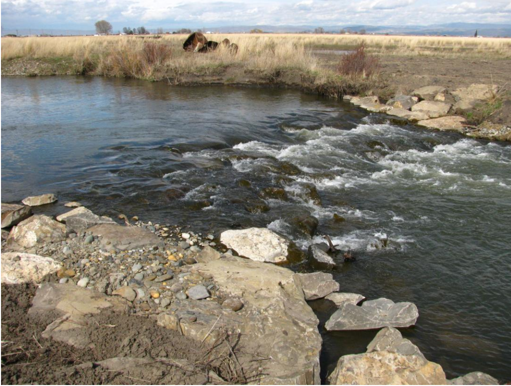
Grade Control Structure in Toppenish Creek
