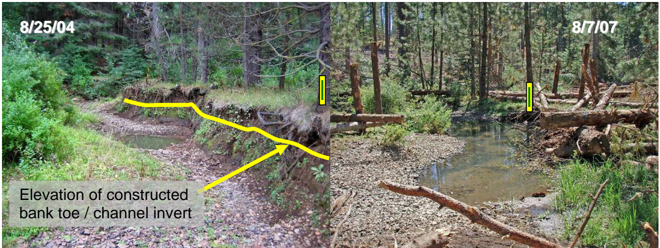
Figure 6. Riffles were filled with gravel to establish new base elevation (Station 6+60).
