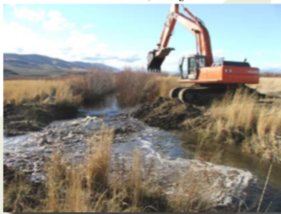
With the grade control structures in place, a backhoe operator breaches a temporary de-watering dam, allowing water from Mid-Toppenish Creek to flow along its historic channel. (Photo courtesy Tracy Hames.)
