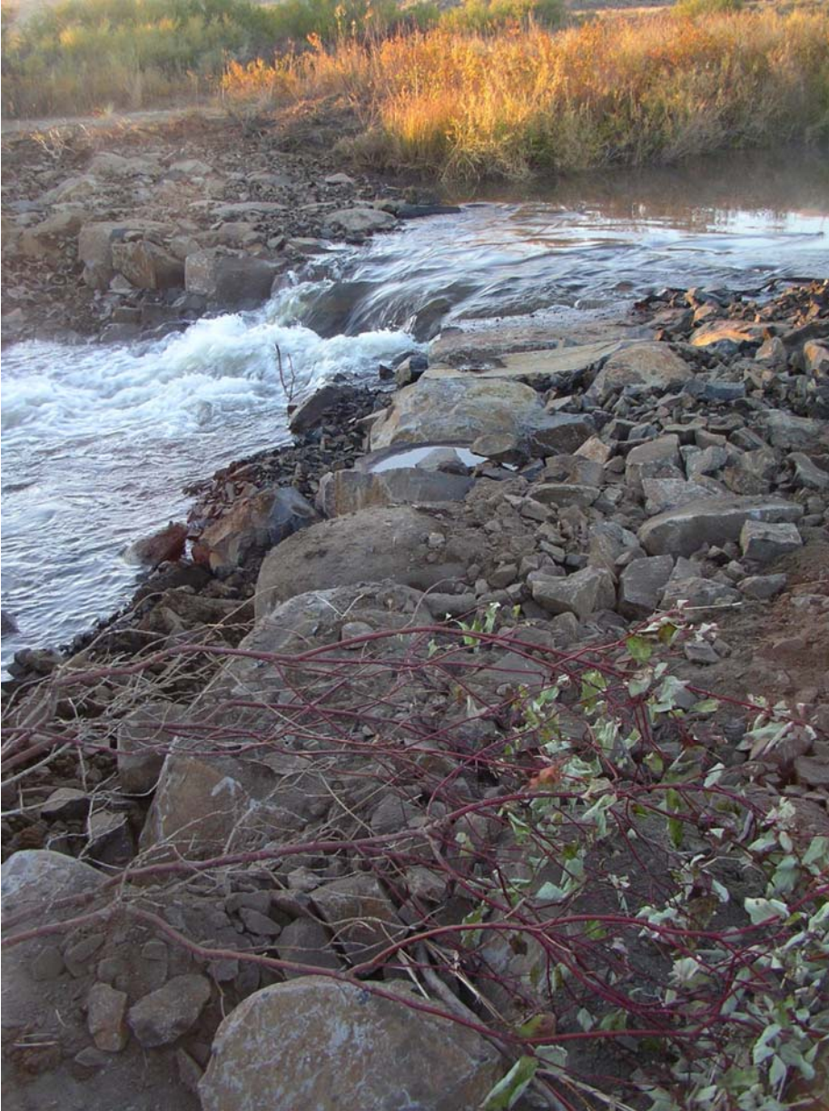
Grade control structure – Mid-Toppenish Creek Restoration Project
