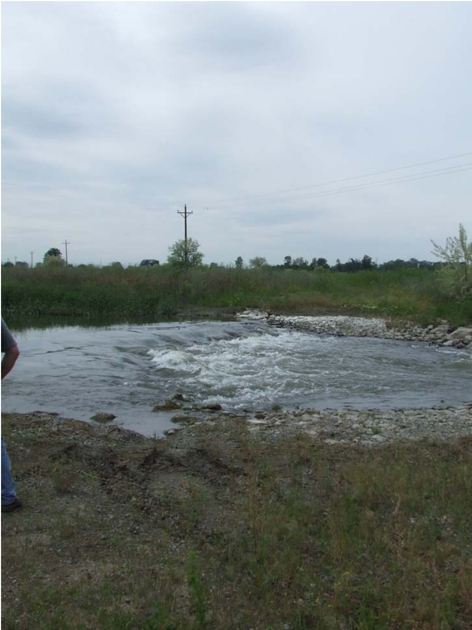
Grade control structure at North Satus Wildlife Area.
