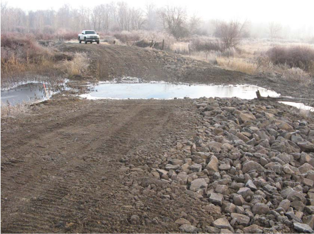
Completed reconnection, Menenick Wildlife Area.
