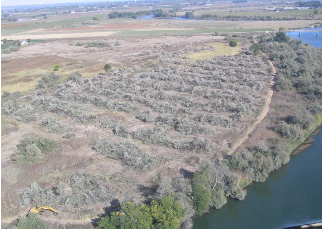
Windrows of Russian olives, removed for the Sulphur Creek Wetland Project. Note excavator in foreground
