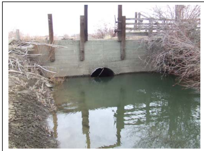
Undersized culvert
