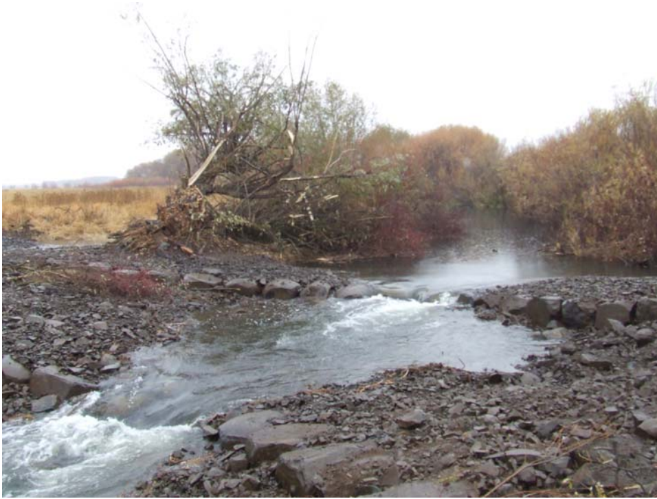
Grade control structure at South Lateral A Wildlife Area.
