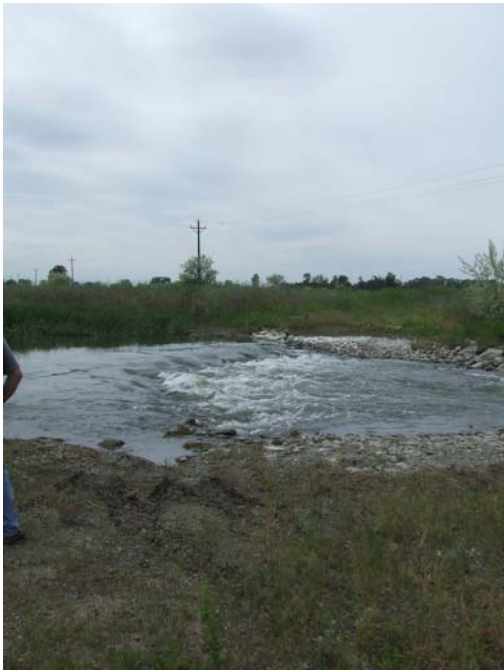
Grade Control Structure installed on North Satus Property
