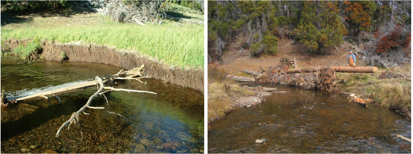
Figure 15. Bank before (7/28/03, left) and after (10/29/04, right) LWD jam construction at Site 4, Element 12a.
