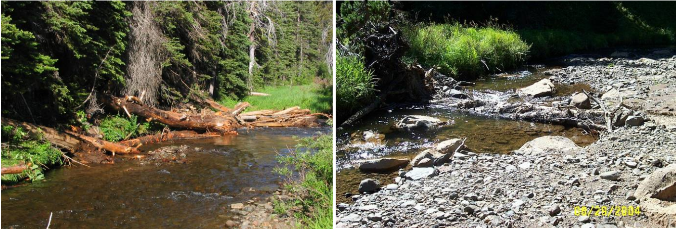
Figure 11. Site 1 as-built photos: LWD jam (element 5, left) and LWD and riffle coarsening at (elements 9 and 10, right).
