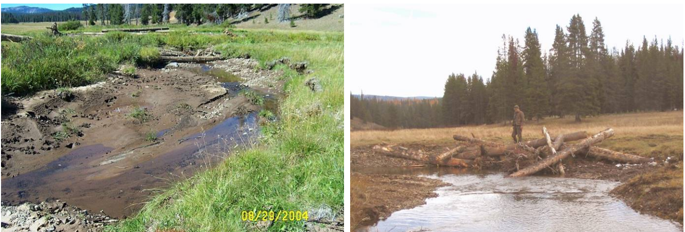
Figure 14. Fine sediment trapped in former avulsion channel (Site 4, Element 5, 8/29/04, left) a week after thunderstorms generated near-bankfull flows and seven weeks after construction. Element 7 (right) as-built following modifications on 10/29/04.
