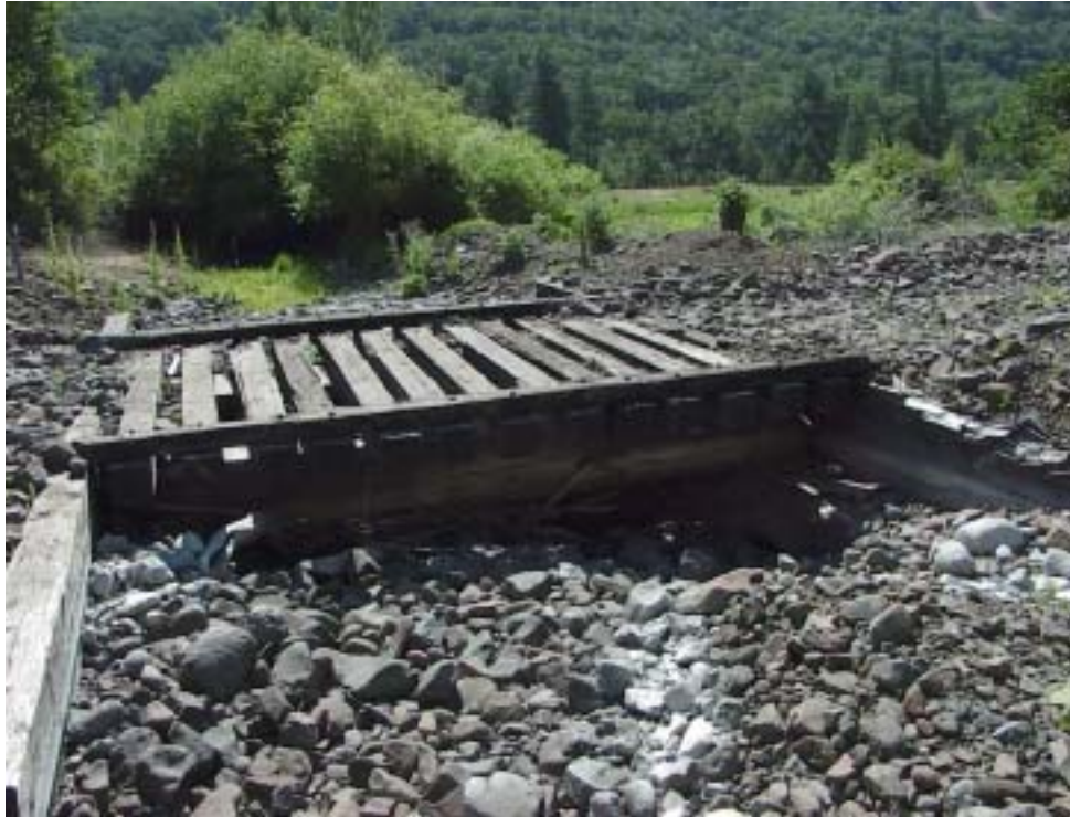
Photo 2. Logging Camp Creek railroad trestle.
