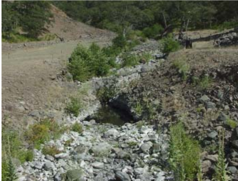
Photo 3. Dillacort Cr. Immediately upstream of Highway 142 crossing.
