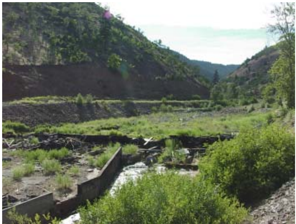
Photo 4. Klickitat mill dam on Snyder Creek.
