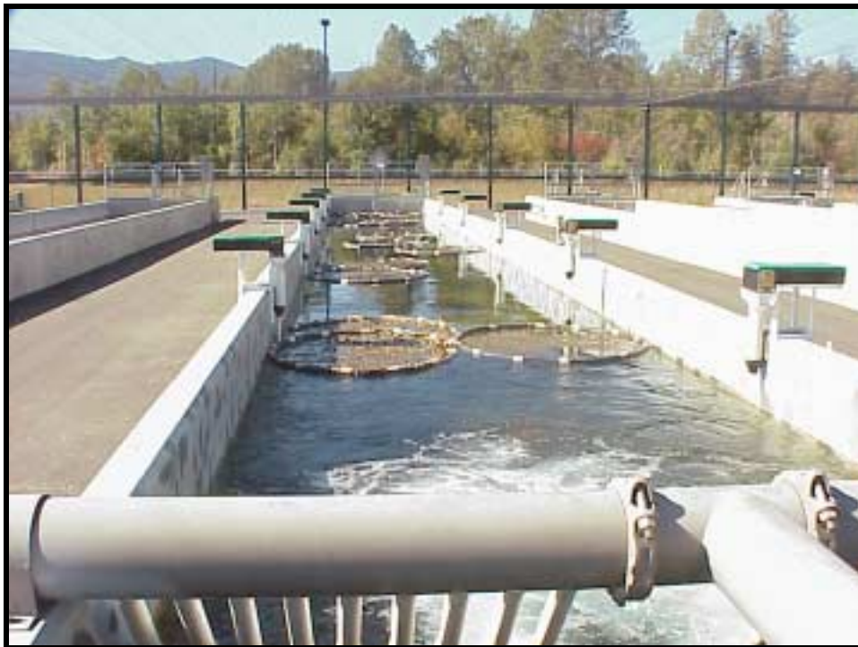
Figure 6. A SNT (semi natural treatment) spring chinook raceway at Cle Elum Supplementation and Research Facility.
