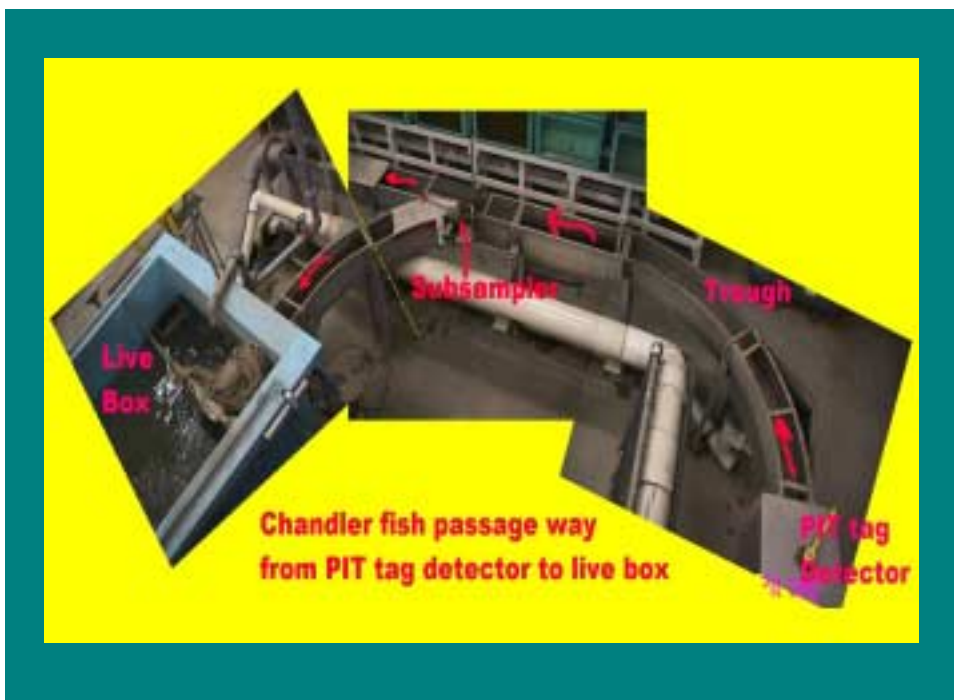
Figure 25. Composite photo depicting the key sampling components at the Chandler Juvenile Monitoring Facility.
