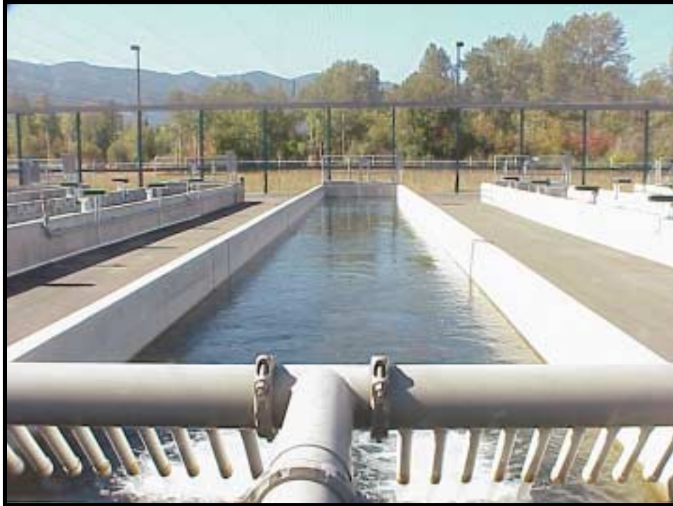
Figure 5. A OCT (optimal conventional treatment) spring chinook raceway at Cle Elum Supplementation and Research Facility.
