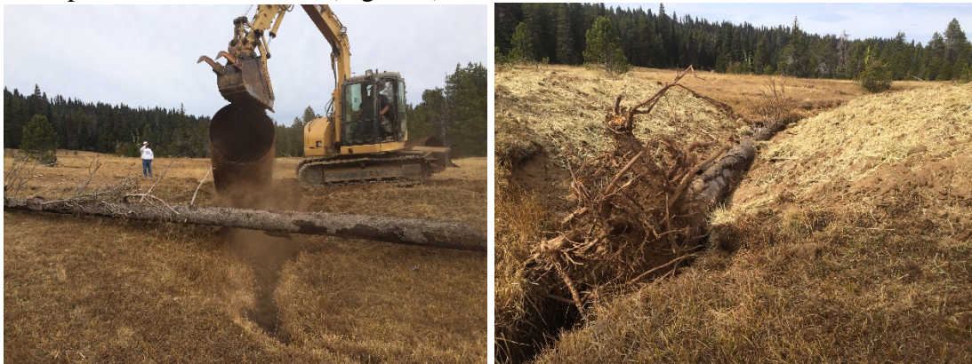
Figure 4 Removal of culver and wind-blown debris with root wad placed in channel
