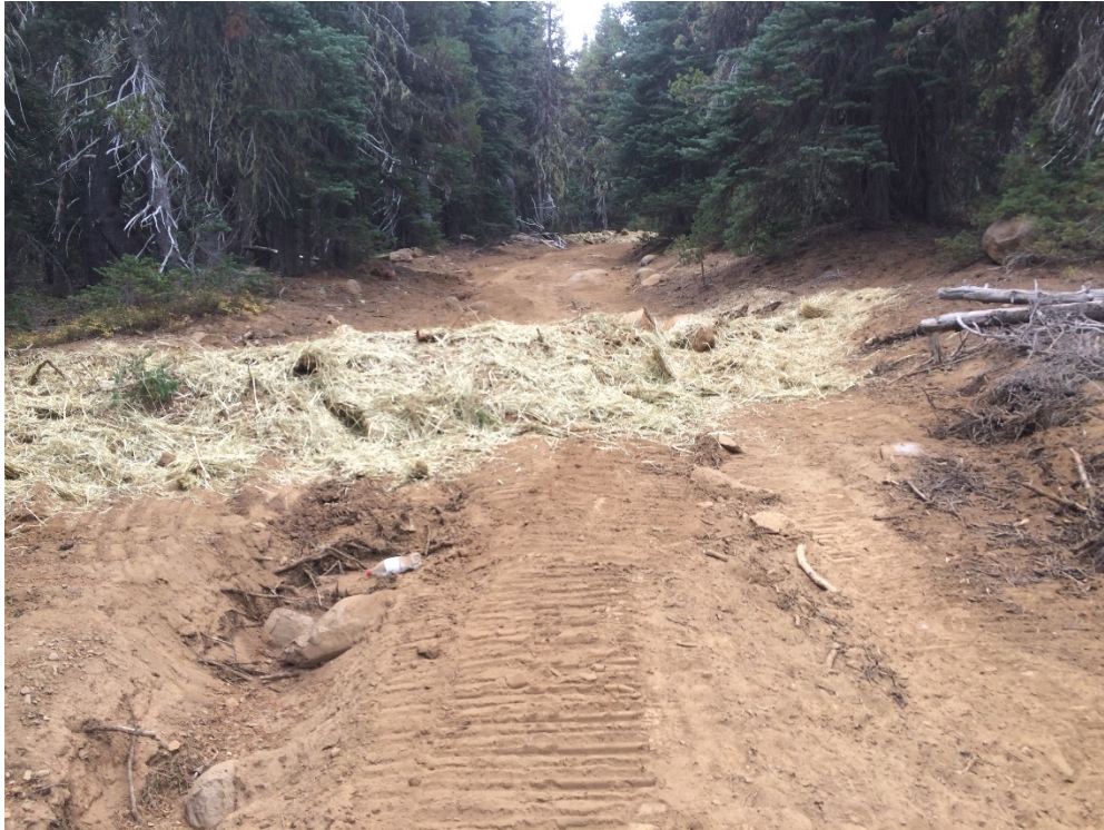
Figure 3 Lakebeds road disturbed areas that was seeded and covered with weed free straw.
