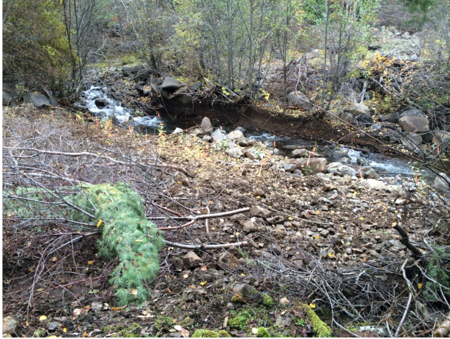
Figure 8. Lower culvert site post construction and revegetation
