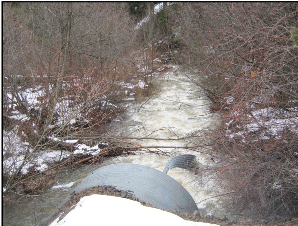
Figure 2. Lower culvert. Photo taken March, 2012
