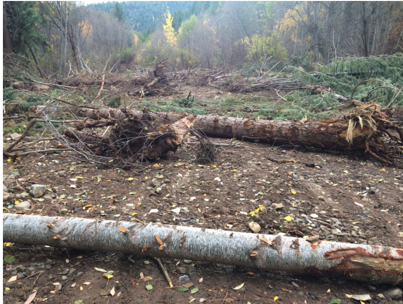
Figure 5. Salvaged logs spread throughout the disturbed area (previous road prism occupation) at the upper culvert site.
