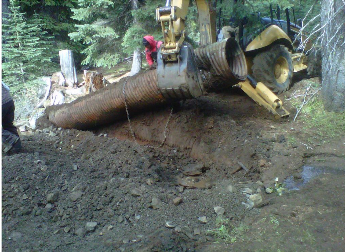
Figure 5. Fish barrier culvert removed.
