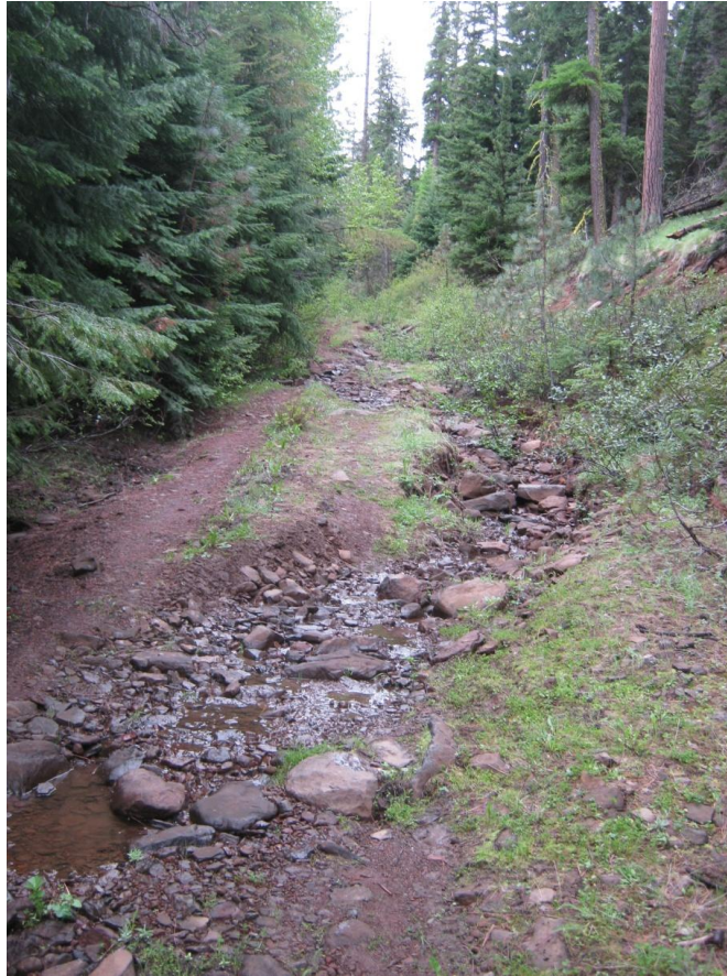
Figure 7. Roadway capturing stream channel pre-treatment.
