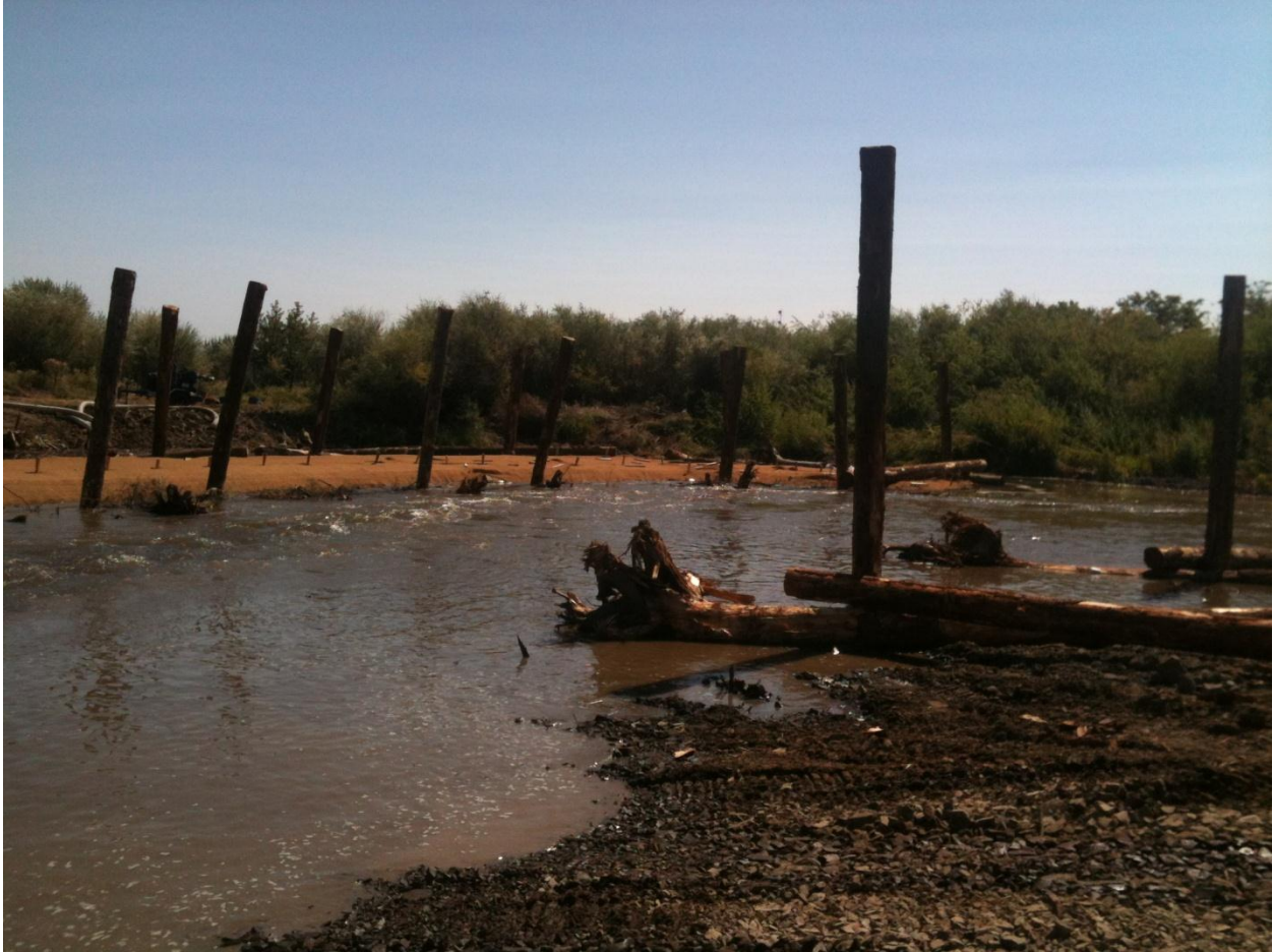
Figure 5. Site response following final coffer dam removal.
