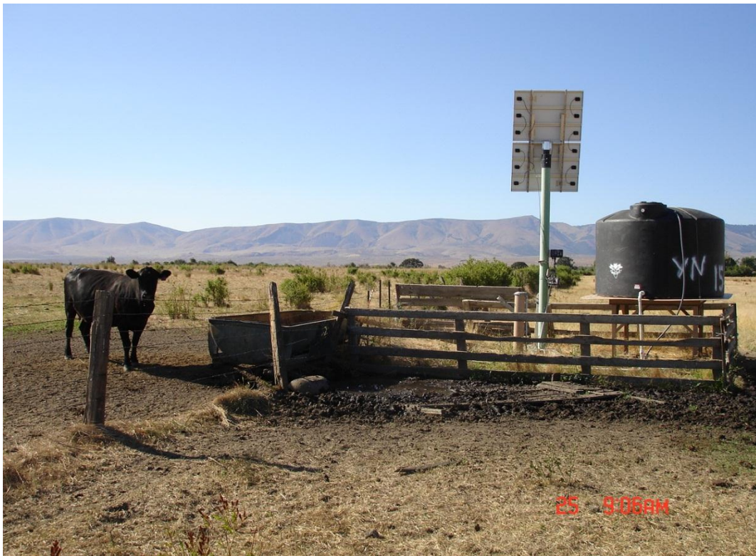
Figure 20. Stock pump and watering trough.
