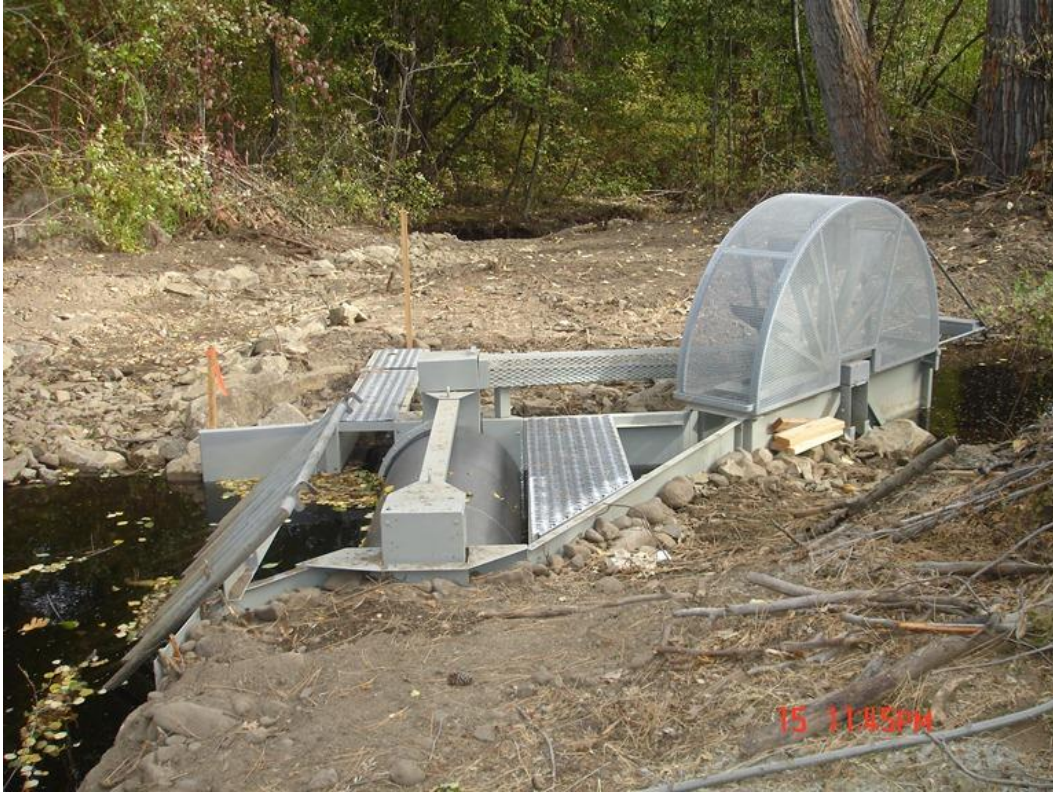
Figure 9. Photo illustrating the South Fork Feeder Fish Screen post-installation
