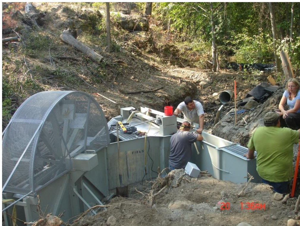
Figure 11. Fish screen installation
