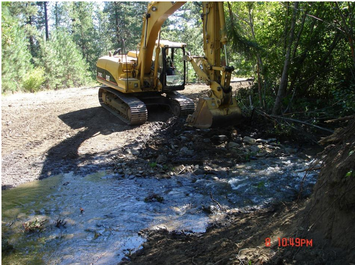
Figure 16. Roughened channel installation post culvert removal
