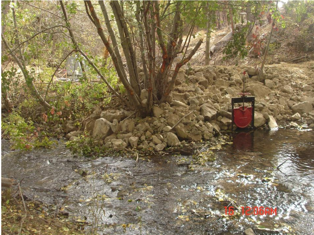
Figure 10. Berm constructed over gated culvert. Note fish screen in background.
