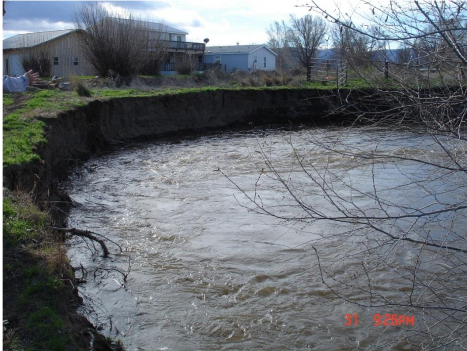
Figure 17. Looking upstream at eroding bank, March 2012
