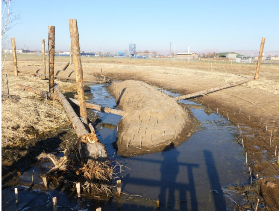
Figure 39. Backwater #1: displaying re-vegetation, woody debris and erosion control measures.
