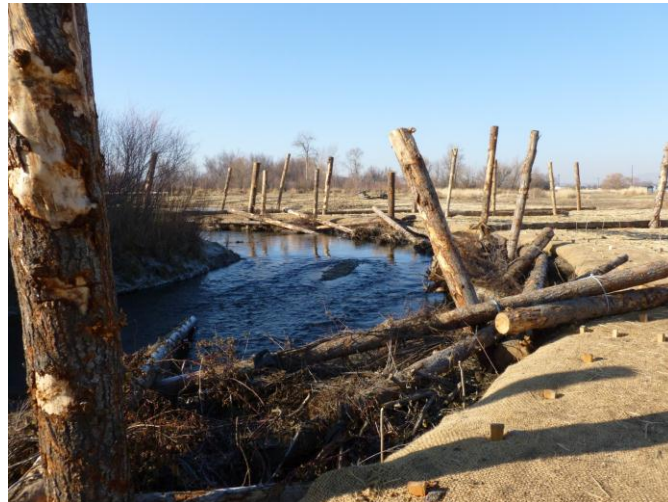
Figure 35. Site #2 post construction
