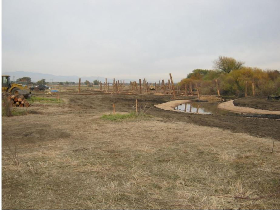
Figure 37. Excavated floodplain, floodplain wood, & backwater #2.
