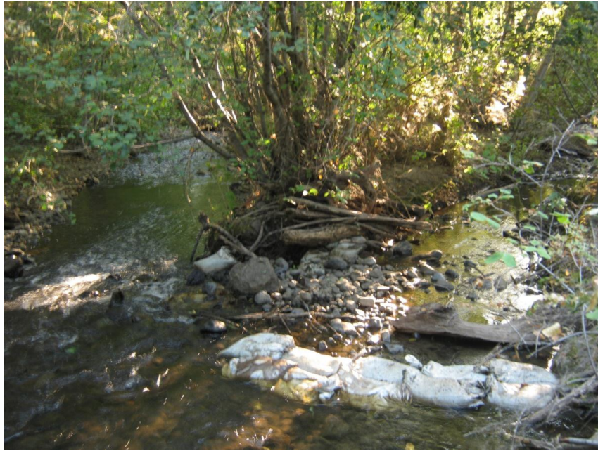
Figure 45. The Feeder Ditch is located on right looking downstream. Sandbagging at the diversion point is to maintain minimum in stream flow.
