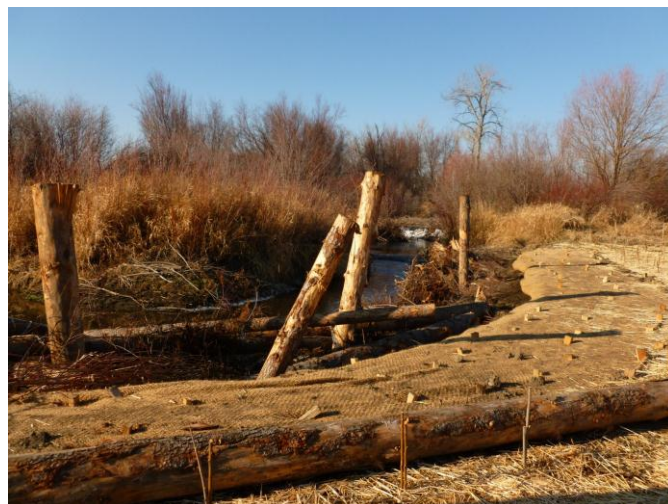
Figure 36. Site # 3 post construction
