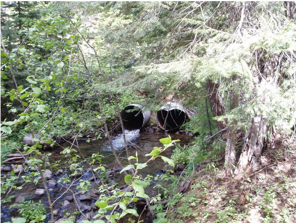
Figure 26. Culvert # 2. Outfall of double culvert configuration at lower Panther Creek
