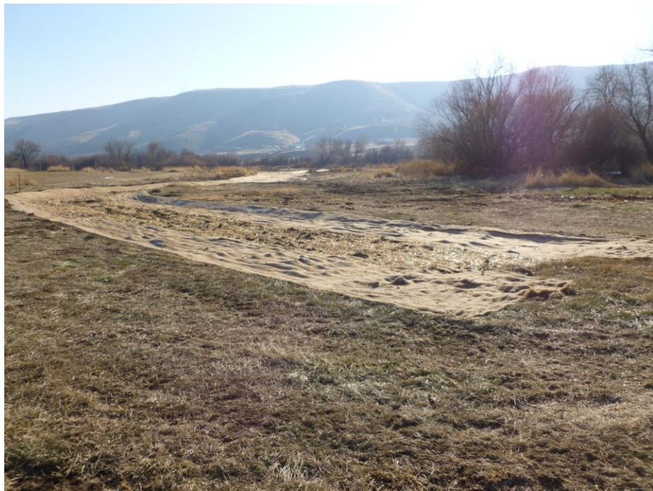
Figure 38. Constructed swale to convey overland flow.
