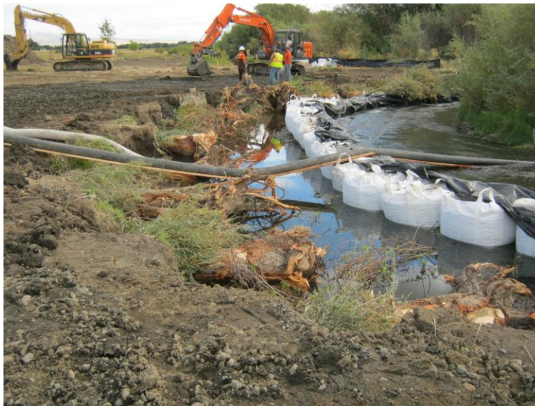
Figure 33. Site #2 during construction.
