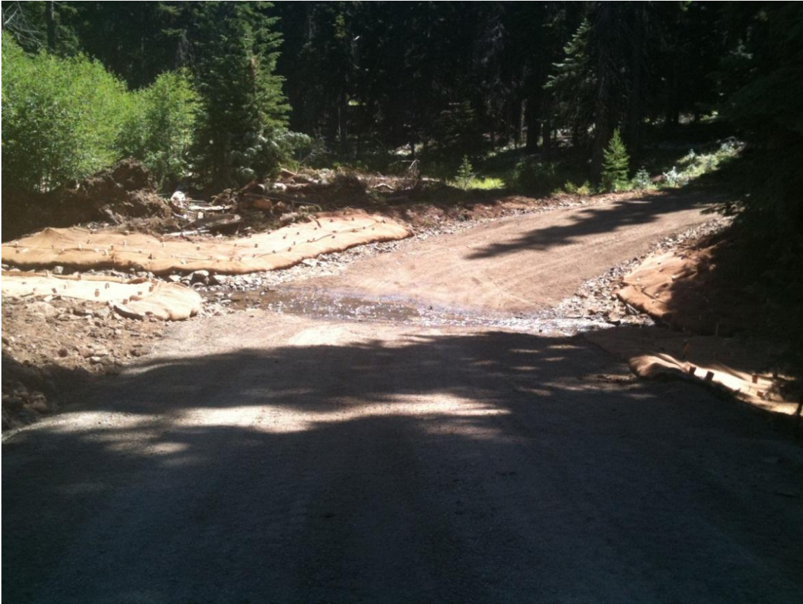
Figure 27. Culvert # 2. Armored rock ford replacing culvert on lower Panther Creek
