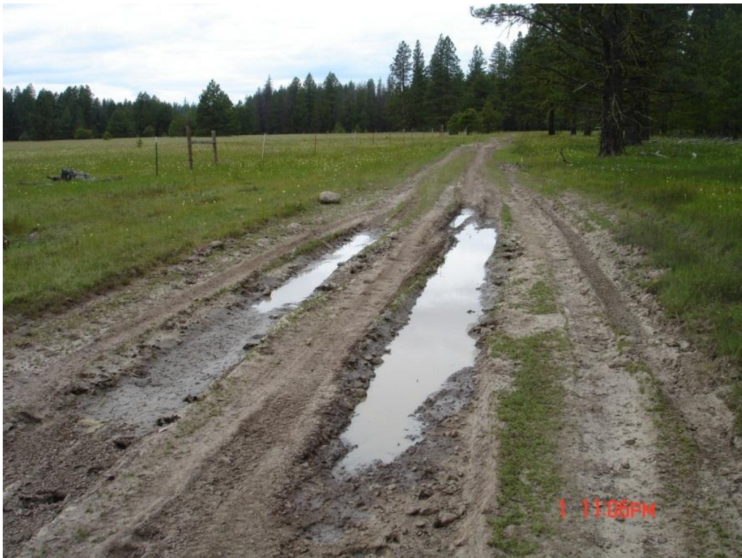
Figure 17. Camas patch meadow located left of picture and road that is widening and channelizing the meadows hydrology.
