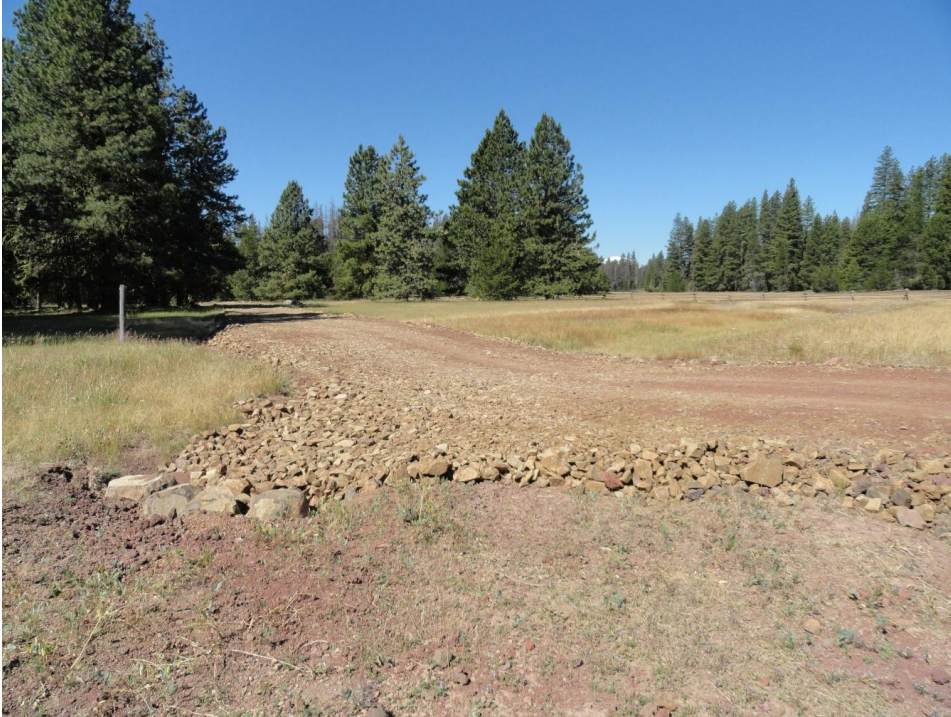
Figure 21. Armored rock ford in place of culvert.
