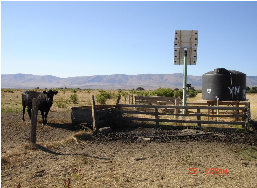
Figure 40. Stock pump and watering trough.
