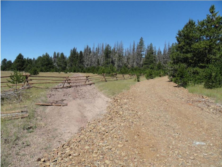
Figure 19. Road closure and road development of alternate route. Also note vehicle exclosure fence to prevent continued use of closed road.
