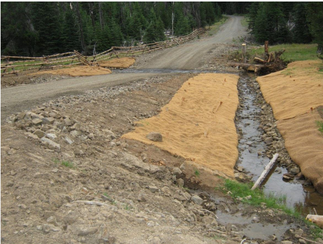
Figure 25. Culvert # 1. Armored rock ford replacing culvert on Rd. 80 crossing
