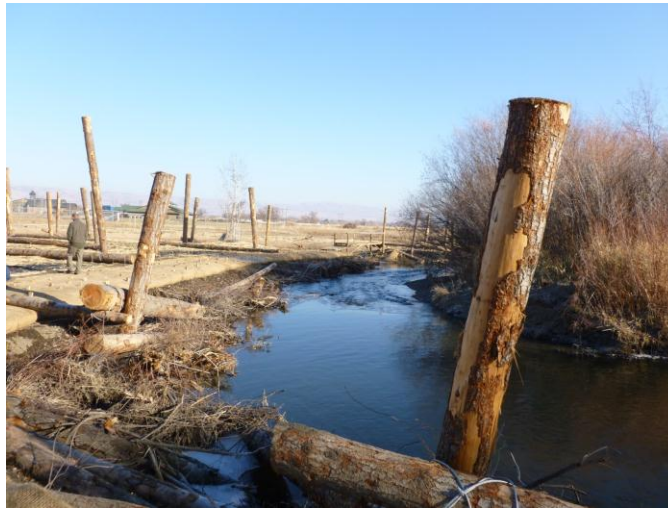
Figure 34. Site #1 post construction
